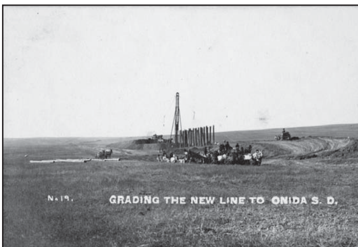
Photo from the S.D. State Archives of the grading portion of a project to Onida, S.D. date unknown
