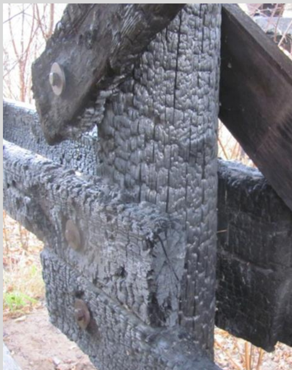
Condition State 3 Fire damage on a timber piling (section loss between less than 10%).
