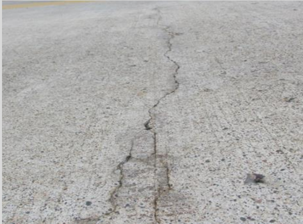
Condition State 3 Transverse crack (1/16" or 0.06" wide) on a bare concrete deck
