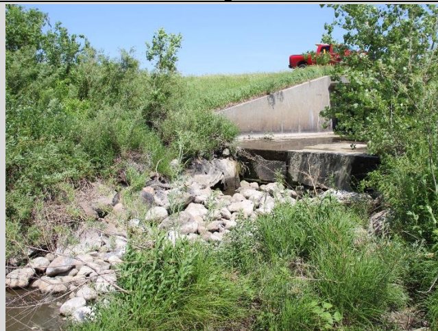
Condition State 3 Scour exceeds tolerable limits at the end of the apron.
