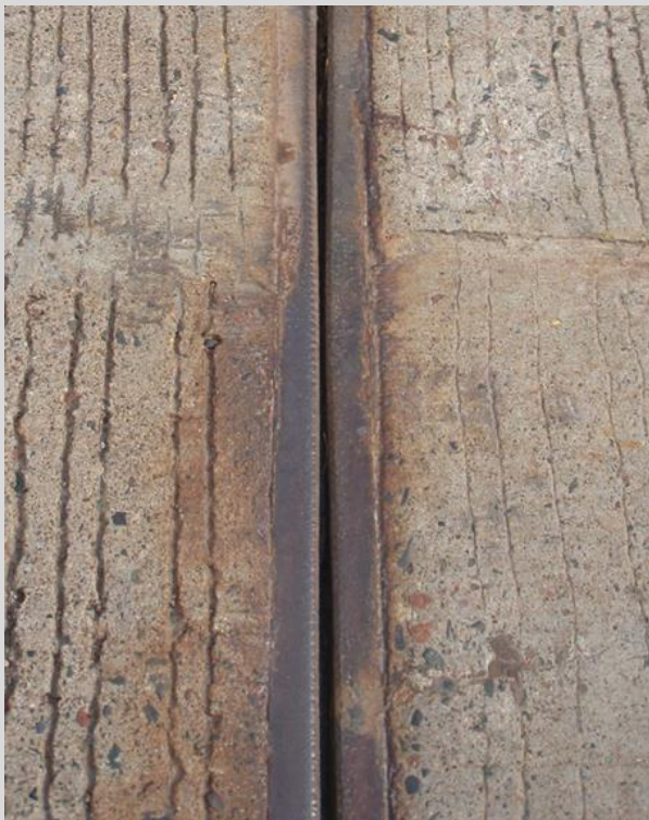
Condition State 3 Strip seal deck joint closed to less than a 1/2" gap
