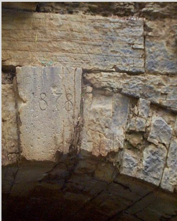
Condition State 2 Weathering (section loss less than 10%) of fascia blocks on a masonry arch culvert.
