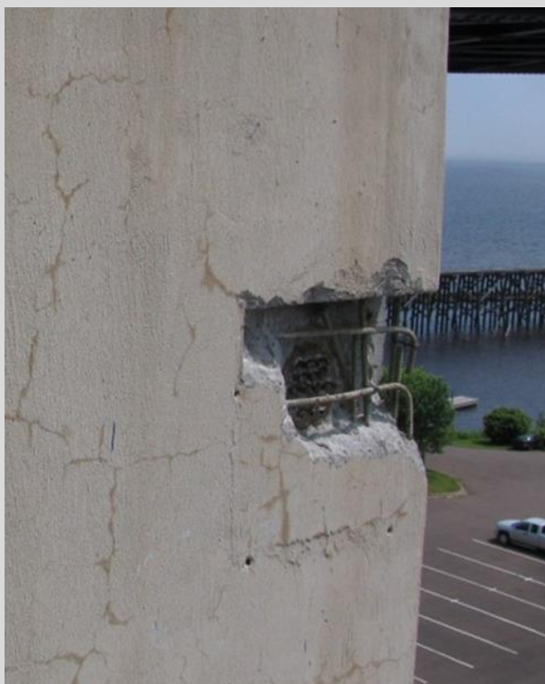
Condition State 3 Spalled end cap on a post-tensioned concrete pier cap.
