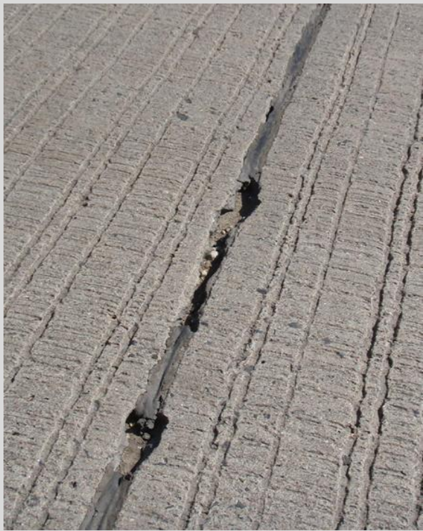
Condition State 3 Section of poured seal missing
