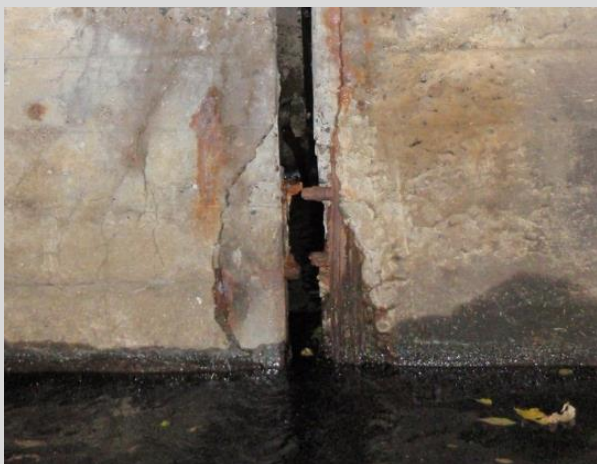
Condition State 3 Severe separation and deterioration at a construction joint on a cast-in-place (CIP) concrete box culvert.
