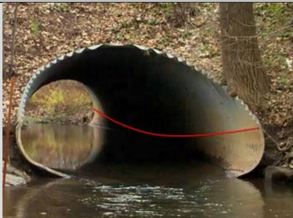
Condition State 3 Significant longitudinal deflection.
