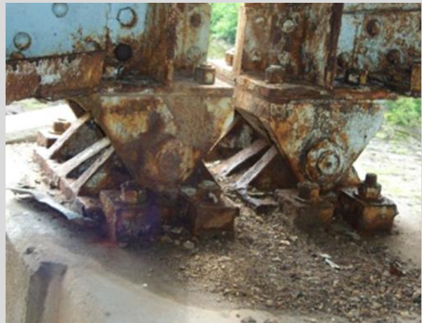
Condition State 3 Flaking rust (section loss) and debris on two fixed pin bearings.
