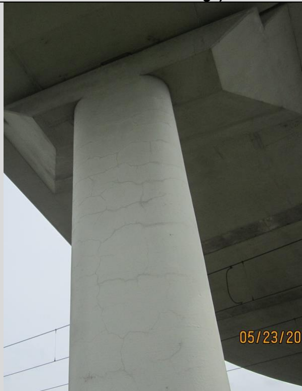
Condition State 2 Moderate map cracking on a reinforced concrete column.
