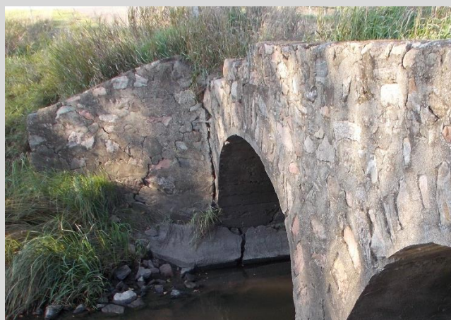
Condition State 3 Extensive crack at the wingwall to barrel connection.
