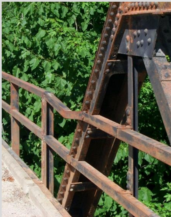
Condition State 3 Steel angle railing bent significantly
