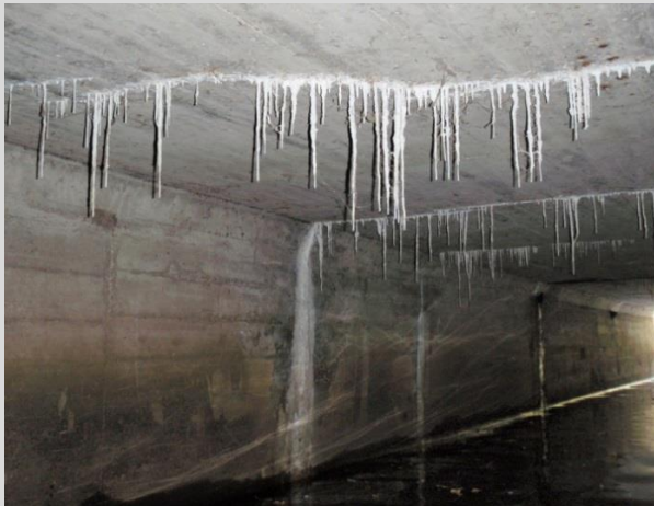
Condition State 3 Heavy leaching on a cast-in-place (CIP) concrete box culvert.
