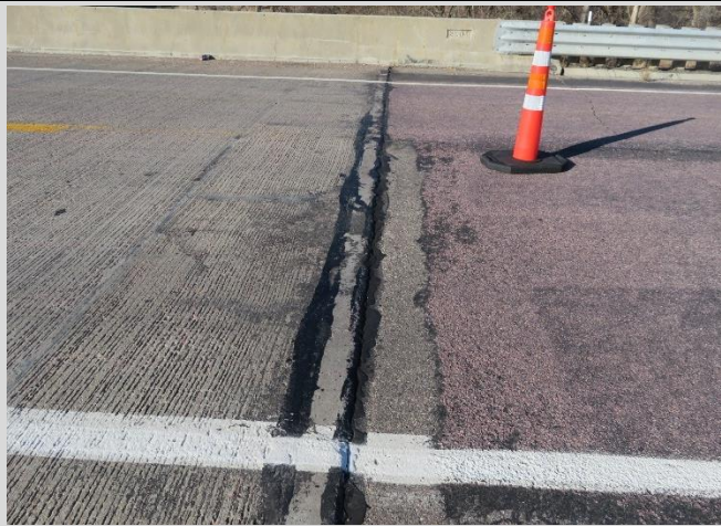
Condition State 2 (Asphalt Approach) Slight to moderate truck movement noted at the end of the bridge.
