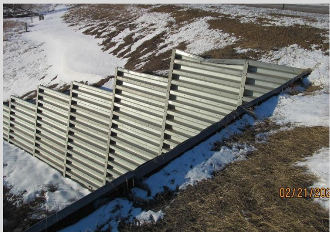
Condition State 2 Damage to the top of a bin wall/wingwall.
