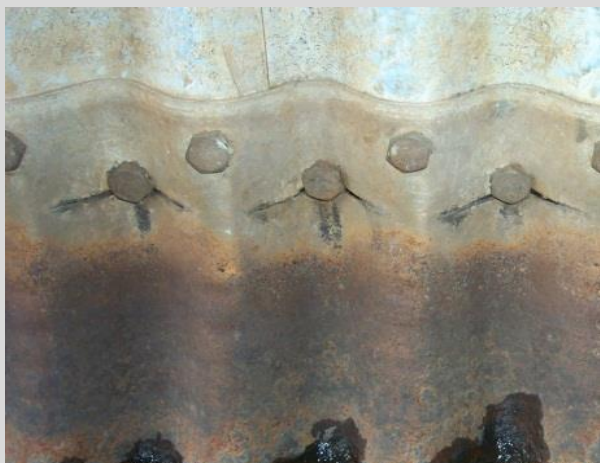
Condition State 3 Cracking along a bolted seam.
