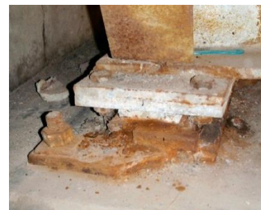
Corroded (possibly frozen) sliding plate bearing
