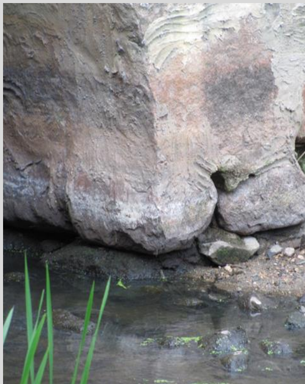
Condition State 3 Scour (mortar missing) along the water line on a masonry arch culvert.
