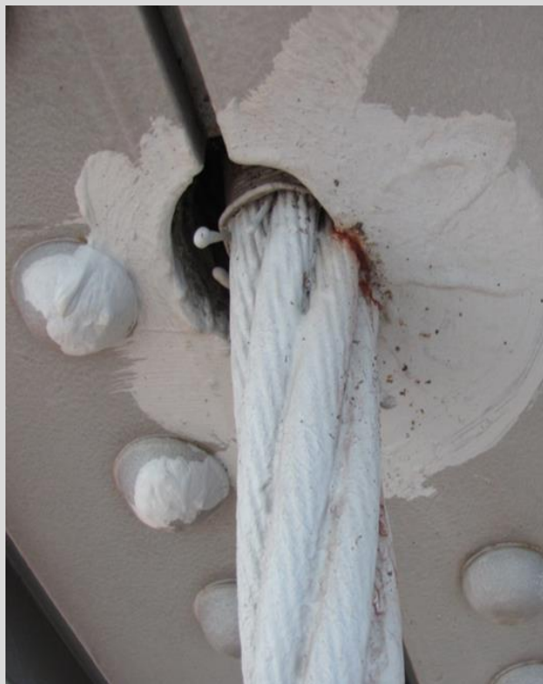
Condition State 3 Active abrasion at contact point (steel wire rope hanger cable wearing against a steel batten plate).
