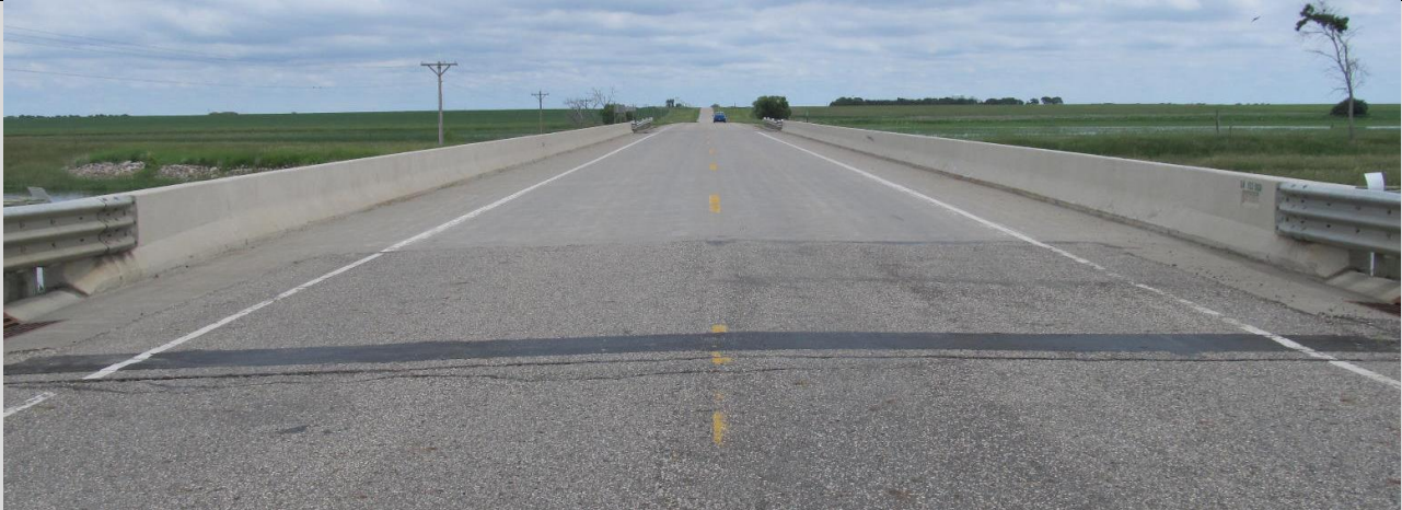
Condition State 2 (Concrete Approach Slab) Slight truck movement and asphalt overlay repair of previously noted significant truck movement and speed reduction.
