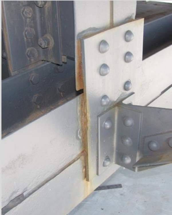
Condition State 3 Pack rust along truss connection
