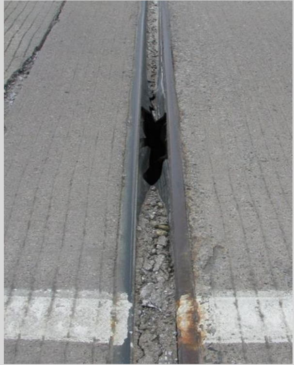
Condition State 4 Hole in strip seal gland
