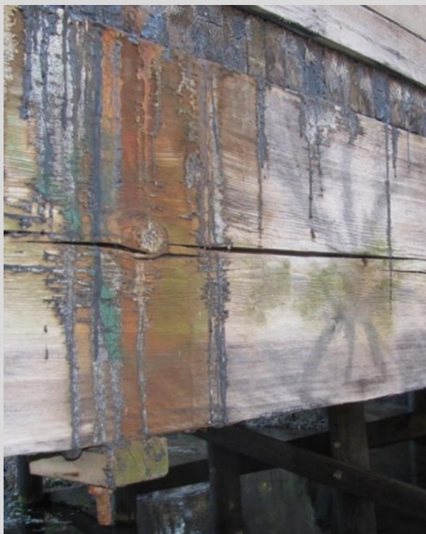
Condition State 3 Significant horizontal splitting on a sawn timber beam.
