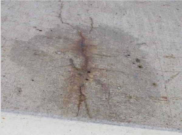
Condition State 3 Map cracked area with rust staining on a bare concrete deck
