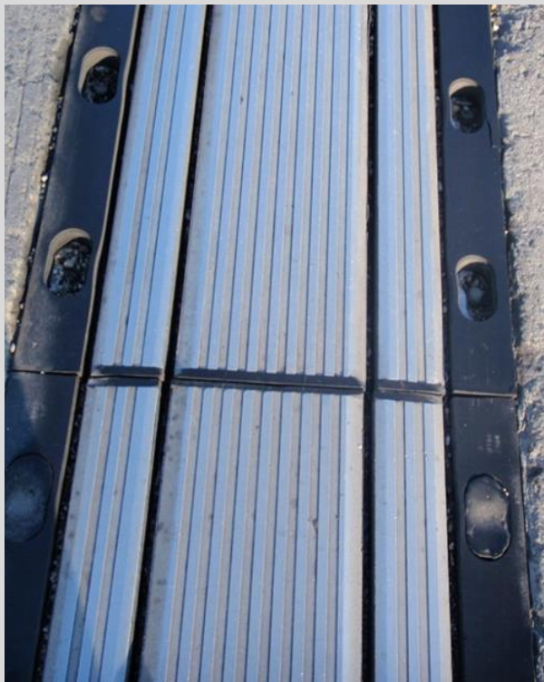
Condition State 2 Anchor bolt covers missing from a “Wabo®Flex” deck expansion joint
