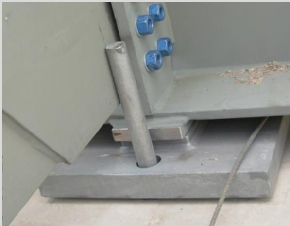
Condition State 3 Improperly installed anchor bolt extends 8" above bearing.
