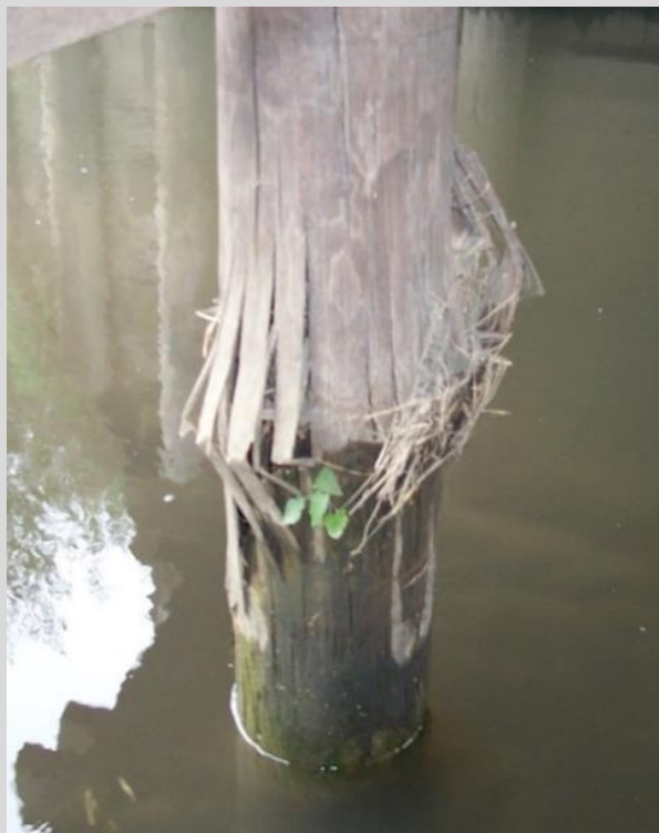
Condition State 4 Timber pile with severe decay and crushing.
