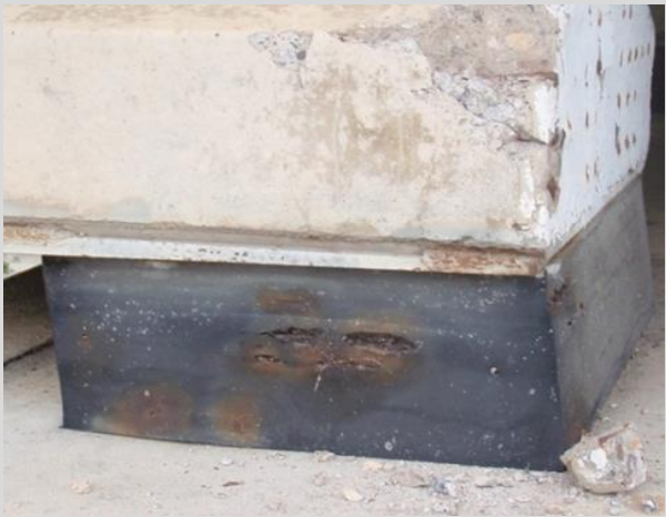
Condition State 3 Pad covering torn, internal plates rusting.
