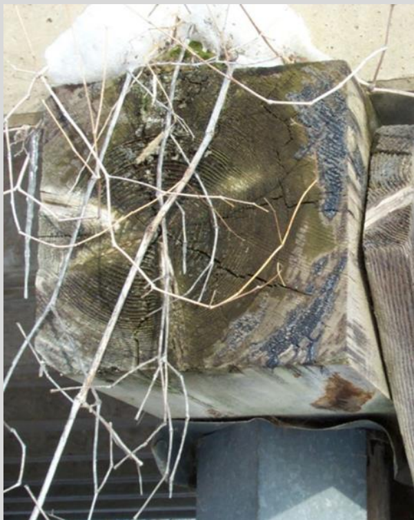
Condition State 2 Checking on the end of a timber pier cap.
