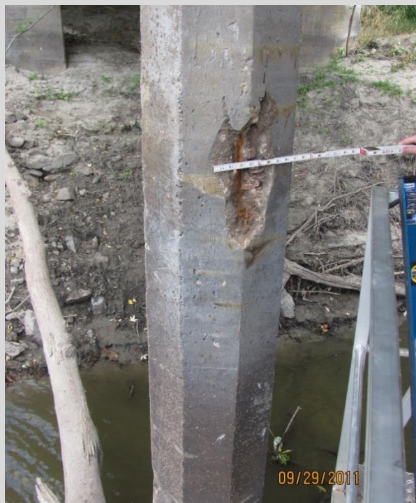
Condition State 3 Significant spall on a precast concrete pile.
