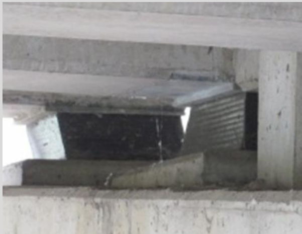
Condition State 2 Elastomeric pads tipped in opposite directions.
