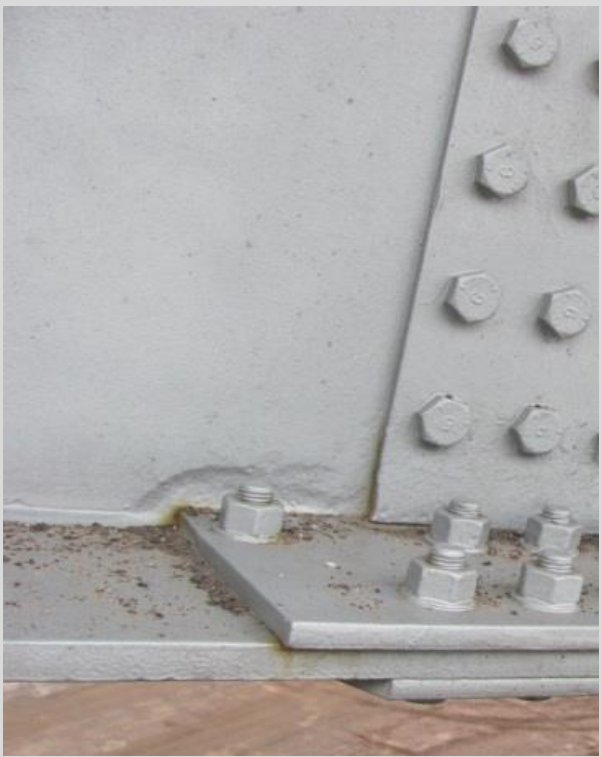
Condition State 3 Pitting in girder web at splice (painted over)
