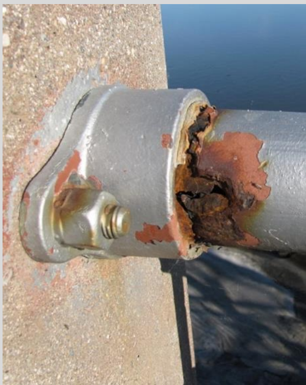
Condition State 4 Horizontal steel rail pipe rusted through at connection to a concrete post
