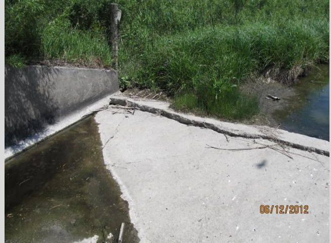
Condition State 3/4 Extensive to severe cracking and deterioration of the cutoff wall to apron connection.
