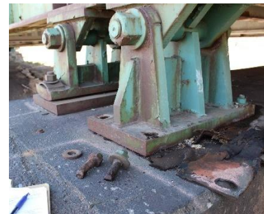
Anchor bolt failure on a fixed bearing
