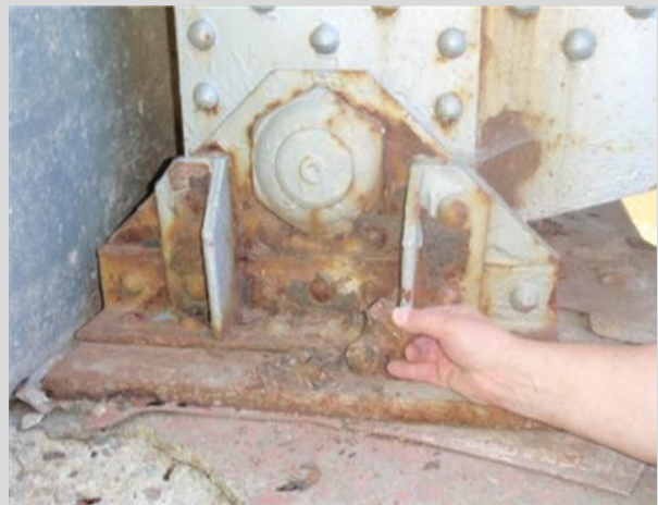
Condition State 4 Anchor bolt failure on a fixed pin bearing (masonry plate has slid back to the parapet).
