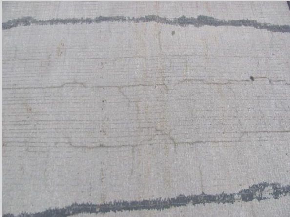
Condition State 2 Map cracking (1/32" or 0.03" wide) on a low slump concrete overlay
