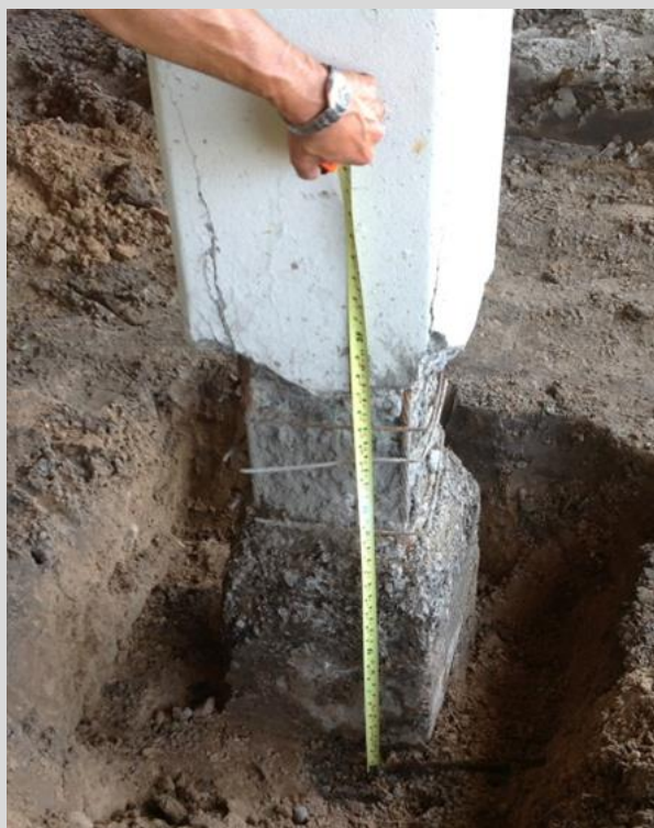
Condition State 4 Severe spalling on a prestressed concrete pile.
