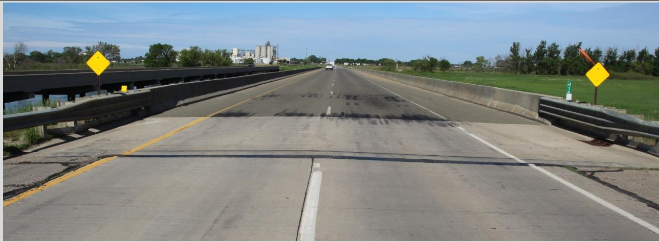
Condition State 4 (Concrete Approach Slab) Significant truck movement, substantial tire bounce/skip markings, bump signs & speed reduction signs in place.
