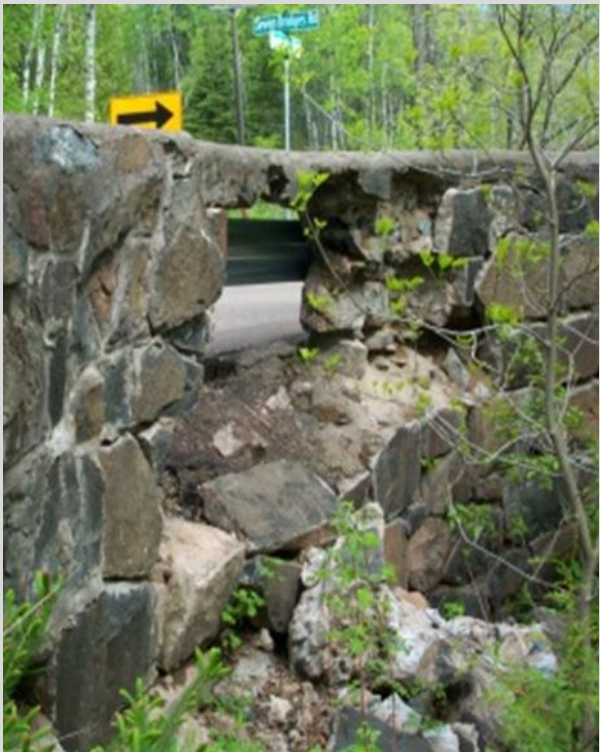
Condition State 4 Severe impact damage on a masonry railing
