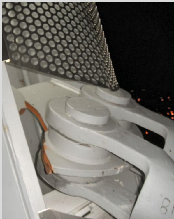
Condition State 4 Cable failure due to fractured anchorage plate.
