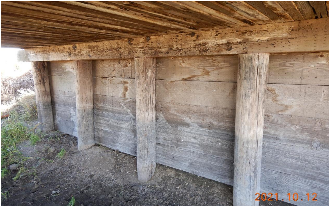
Timber Pier Cap at an Abutment
