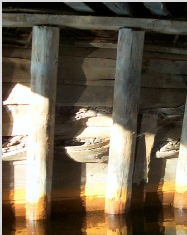
Condition State 4 Failure of abutment backing planks.
