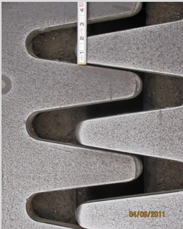
Condition State 3 Finger joint laterally misaligned (fingers contacting)
