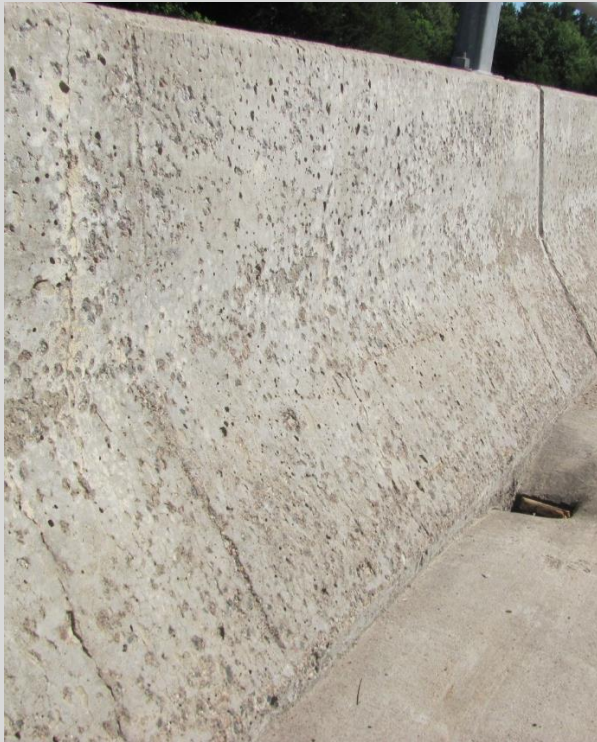
Condition State 2 Scale on a concrete jersey barrier
