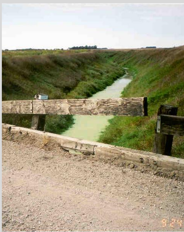
Condition State 4 Timber rail beam detached from posts
