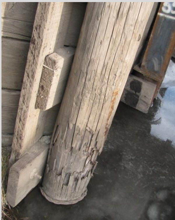
Condition State 3 Shell damage on a timber piling (section loss less than 10%).
