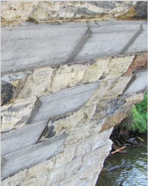
Condition State 2 Concrete repairs on a masonry arch.
