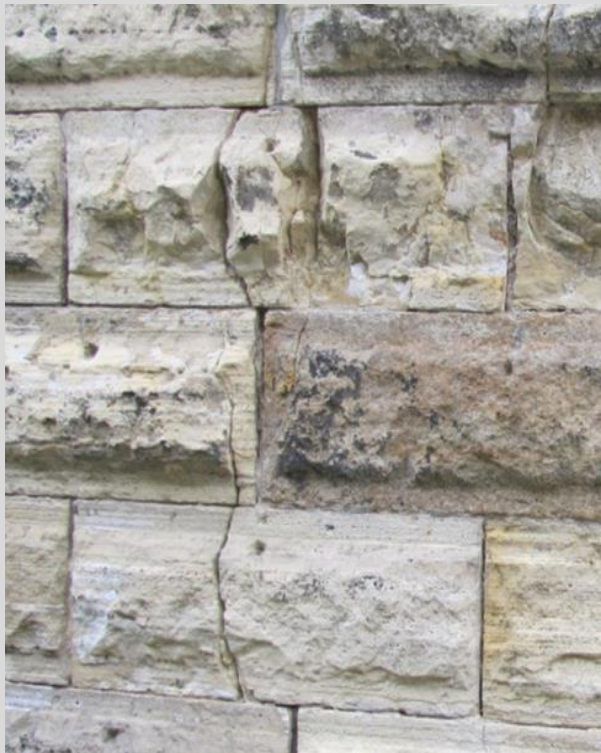
Condition State 3 Fracture in a masonry block continuing into adjacent courses.
