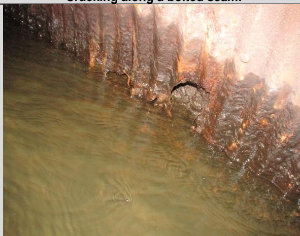
Condition State 3 Through corrosion along the water line.
