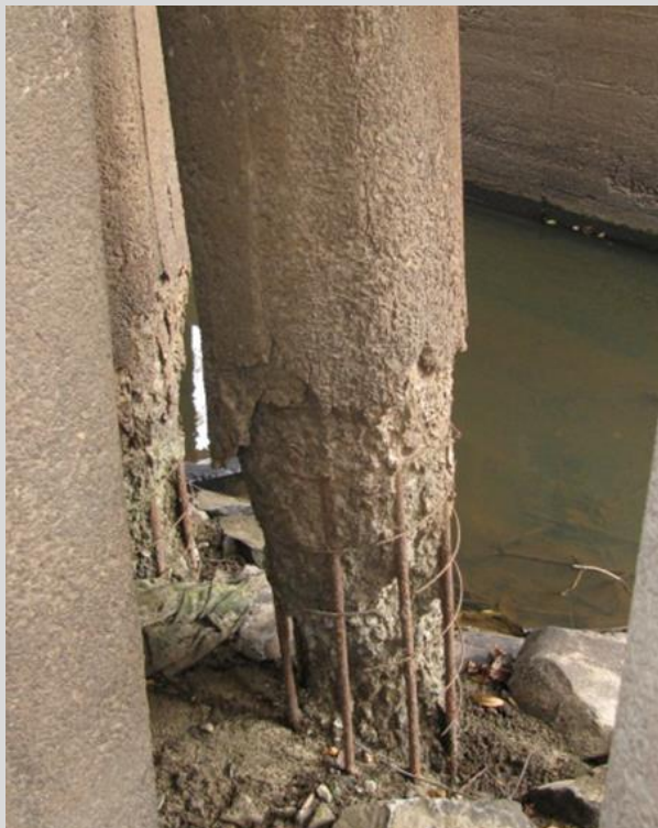
Condition State 4 Severe scale/spall on a reinforced concrete pile.
