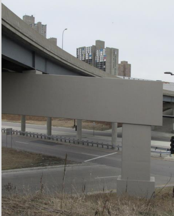
Condition State 1 Post-tensioned pier cap with no defects.
