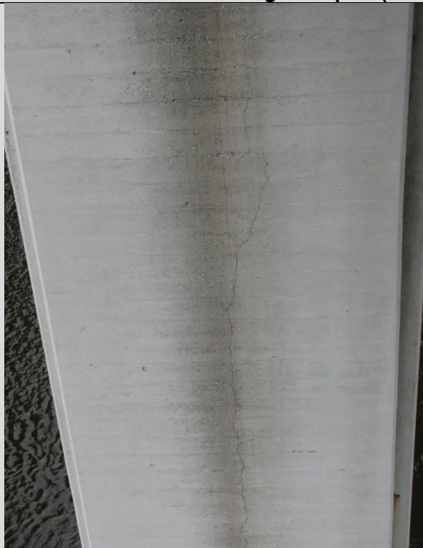
Condition State 2 Moderate width vertical crack on a reinforced concrete column.
