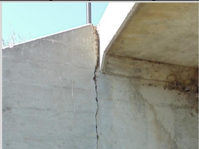
Condition State 3 Extensive cracking/significant spalling at the wingwall to parapet connection.
