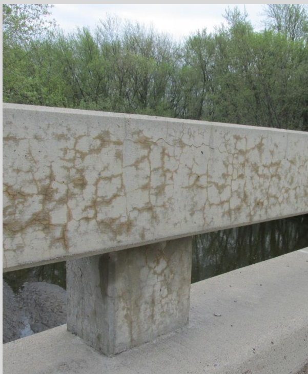
Condition State 2/3 Map cracking on a concrete post & beam railing
