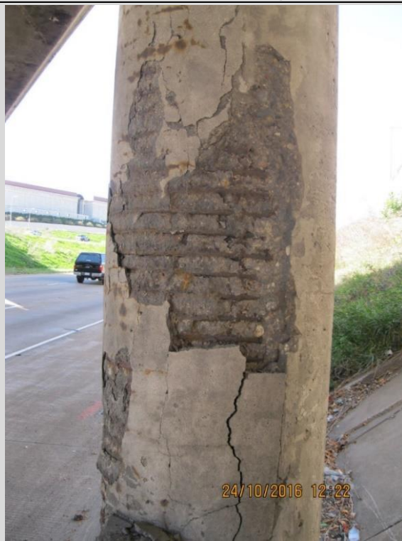
Condition State 4 Extensive spalling (exposed and corroded reinforcement) on a reinforced concrete column.
