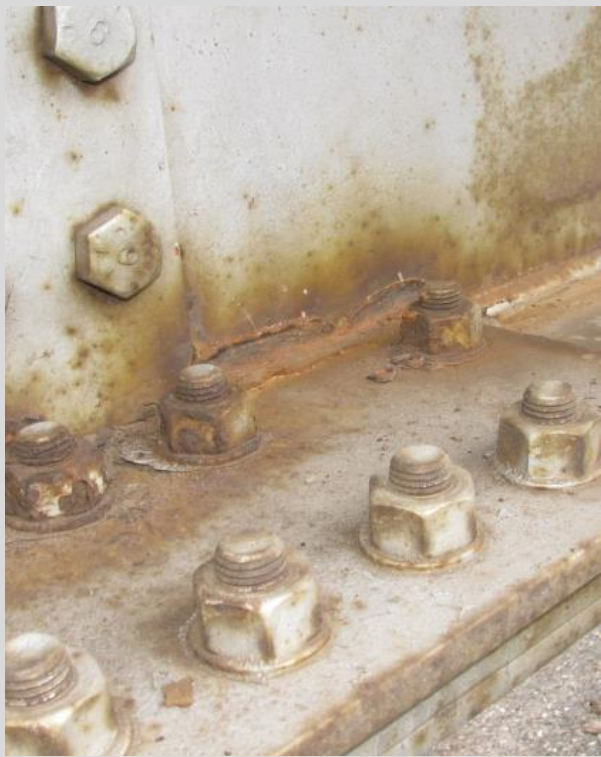
Condition State 3 Flaking rust (and pitting) in girder web at splice
