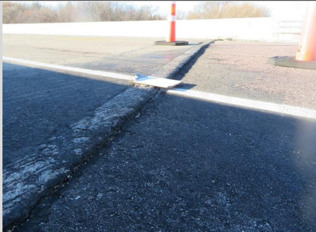
Condition State 3 (Asphalt Approach) Significant truck movement noted at the end of the bridge.
