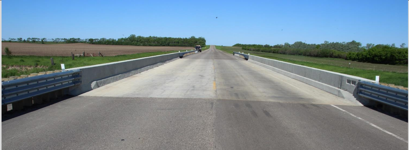
Condition State 2 (Asphalt Approach) Slight to moderate truck movement noted and minimal tire bounce/skip marks at the beginning/end of the bridge.
