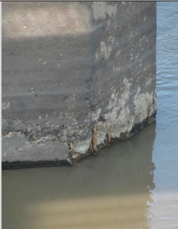
Condition State 3 Significant scale/abrasion along the waterline on a reinforced concrete column.
