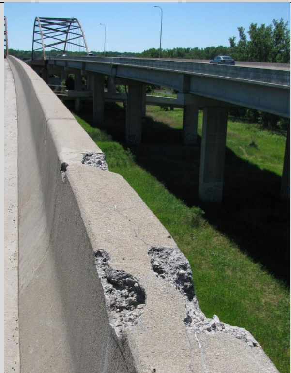
Condition State 3 Spalling/scaling along the top of a concrete jersey barrier
