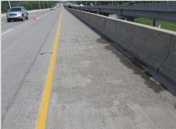
Condition State 2 Scaling (1/4" deep) on a low slump overlay
