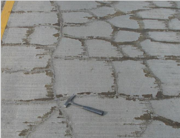
Condition State 3 Map cracking (1/16" or 0.06" wide) with failed sealant on a low slump overlay
