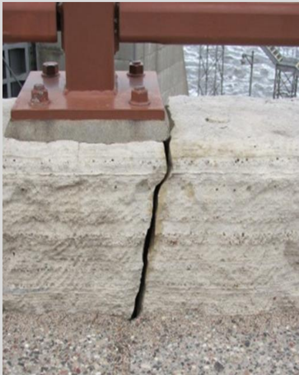
Condition State 3 Block split on a masonry parapet
