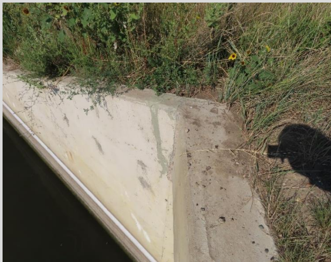
Condition State 2 Repair of a wingwall to parapet connection.
