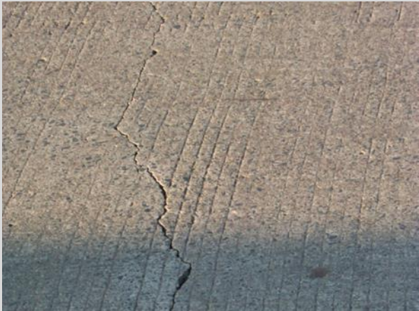
Condition State 3 Crack (1/16" or 0.06" wide) in a low slump overlay
