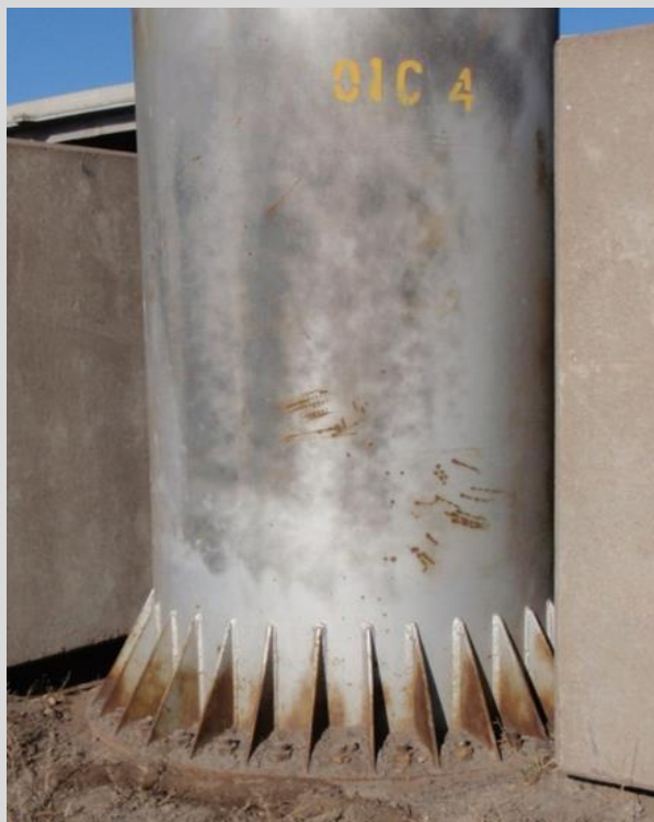
Condition State 2 Paint failure and surface corrosion on a steel column
