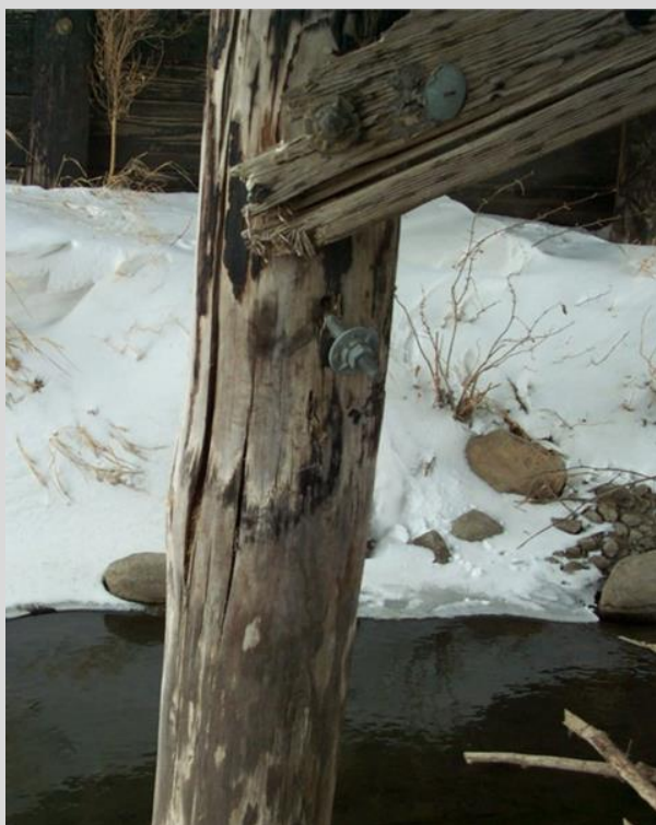
Condition State 3 Timber pile with splitting and decay at a bracing connection.
