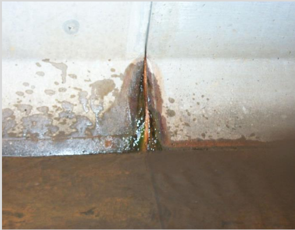
Condition State 2 Minor joint separation/backfill infiltration in-between the segments of a precast box culvert.
