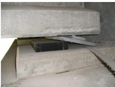
Severe malfunction of an elastomeric bearing
