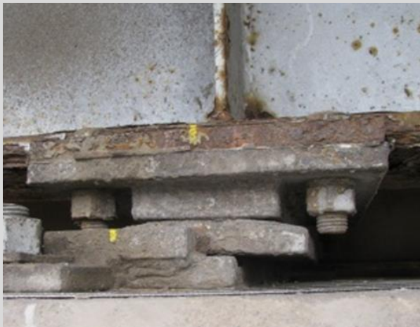
Condition State 3 Sliding plate bearing near expansion limits (slide plate extends well beyond the masonry plate).
