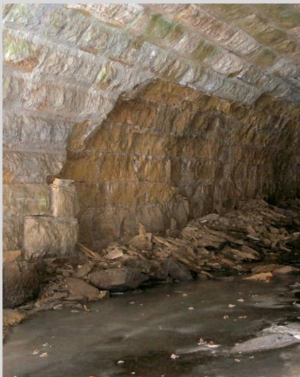
Condition State 4 Severe (and extensive) spalling on a masonry arch culvert.
