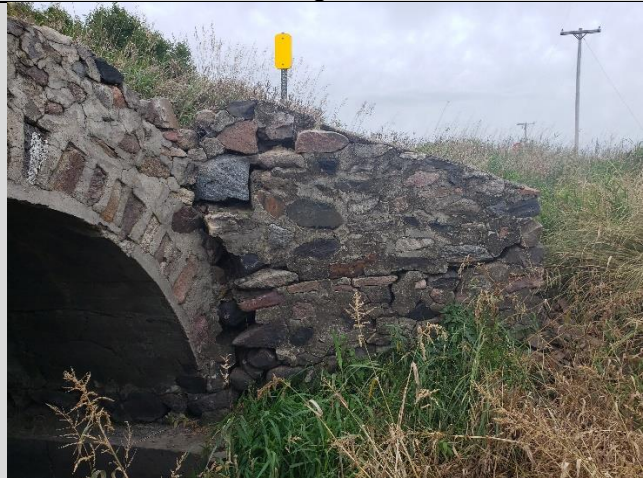
Condition State 4 Severe cracking, spalling, and deterioration of the wingwall.
