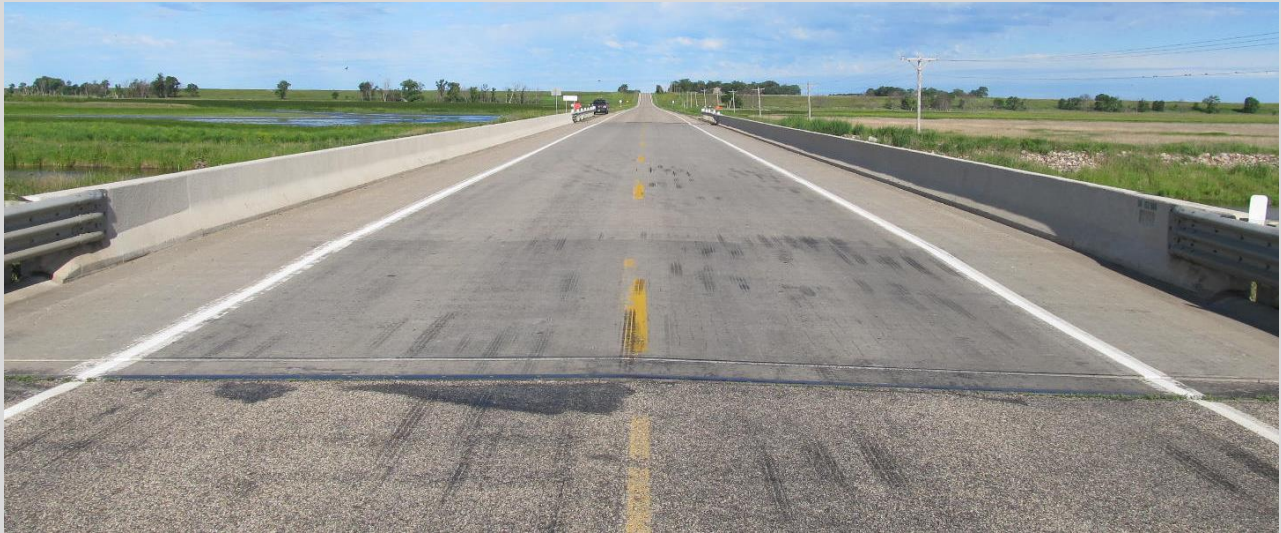
Condition State 3 (Concrete Approach Slab) Significant truck movement, substantial tire bounce/skip markings, slight speed reduction.
