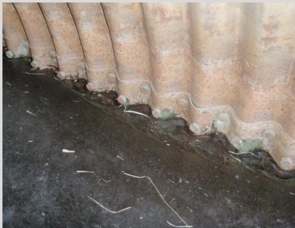
Condition State 2 Surface corrosion along the waterline.
