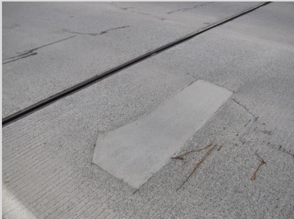
Condition State 2 Sound concrete patch on a low slump overlay
