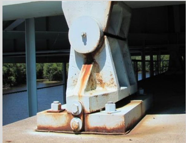
Condition State 2 Surface corrosion on a rocker expansion bearing.
