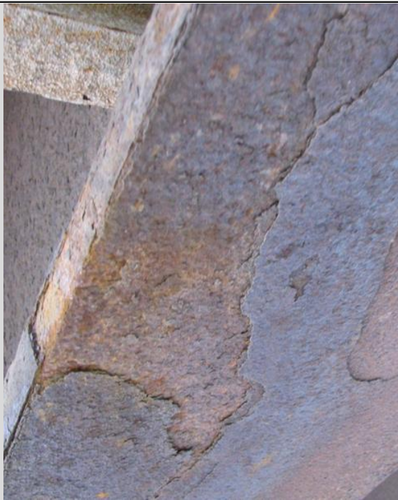
Condition State 4 Weathering steel patina has failed – large areas of surface layer flaking off.
