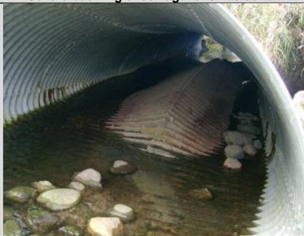
Condition State 4 Severe barrel distortion.
