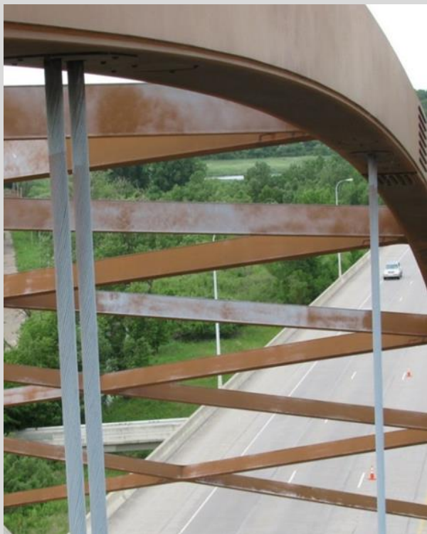
Condition State 2 Chalking paint on steel arch bracing members.
