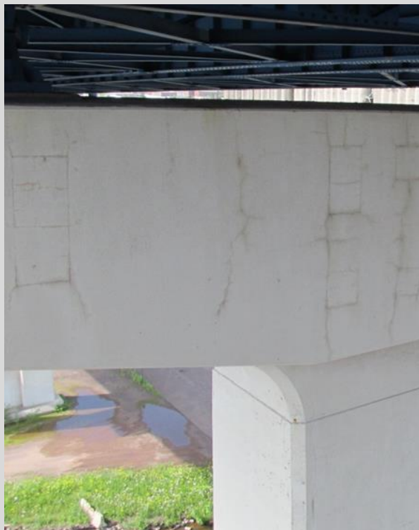
Condition State 2 Cracking on the face of a post-tensioned pier cap.
