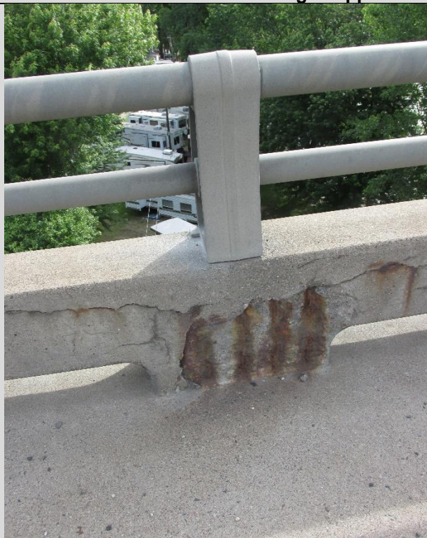
Condition State 3 Spalling and exposed rebar on the concrete parapet of a combination railing
