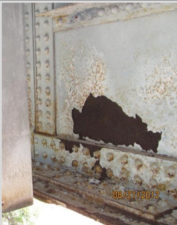
Condition State 4 Paint system failure (exposed steel).
