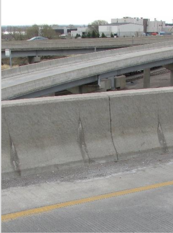
Condition State 2 Vertical cracks with light leaching in a concrete jersey barrier
