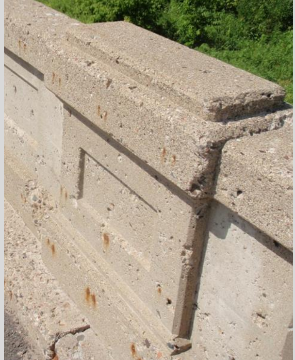
Condition State 2 Scale and pop-outs on a concrete parapet railing
