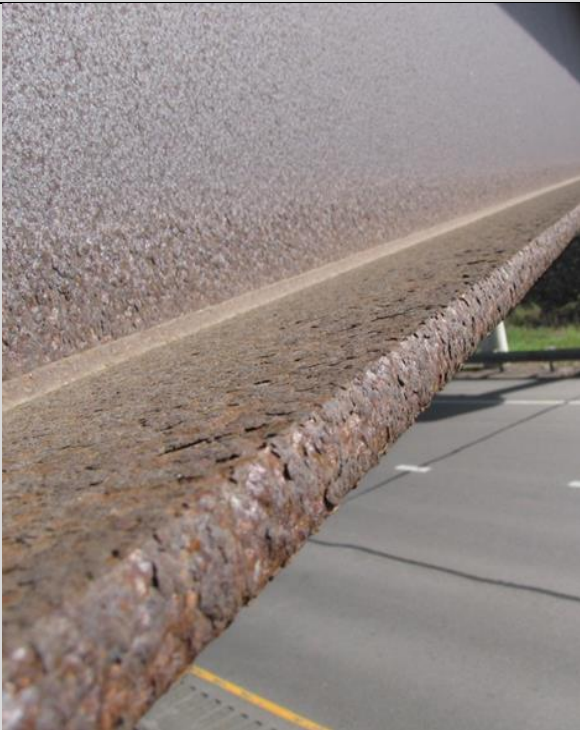
Condition State 3 Weathering steel patina has flaking (less than 1/2" diameter) along the bottom flange.
