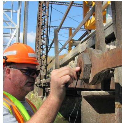
Ultrasonic Examination of a Pinned Truss Connection
