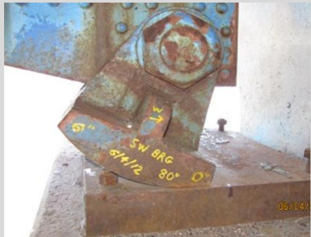
Condition State 4 Rocker bearing locked and sliding on the masonry plate.
