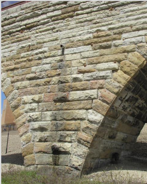
Condition State 2 Staining and scaling (minor section loss) on a masonry arch.
