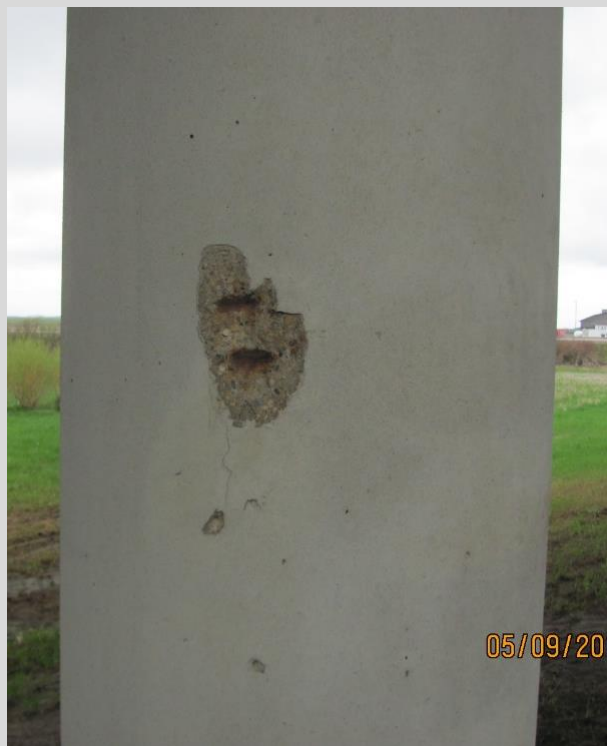
Condition State 2 Isolated spall with exposed reinforcement on a reinforced concrete column.
