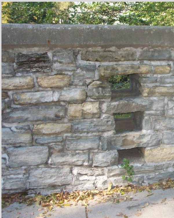
Condition State 2 Minor mortar breakdown on a masonry bridge railing
