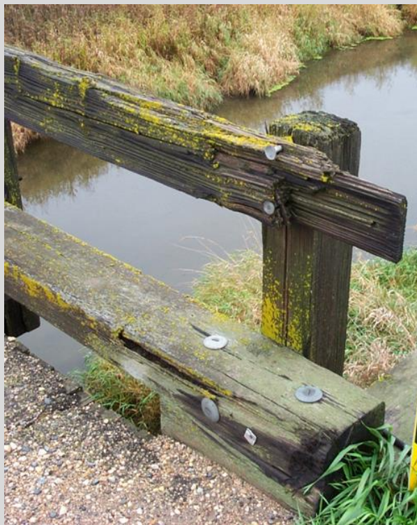
Condition State 3 Significant decay on a timber rail beam
