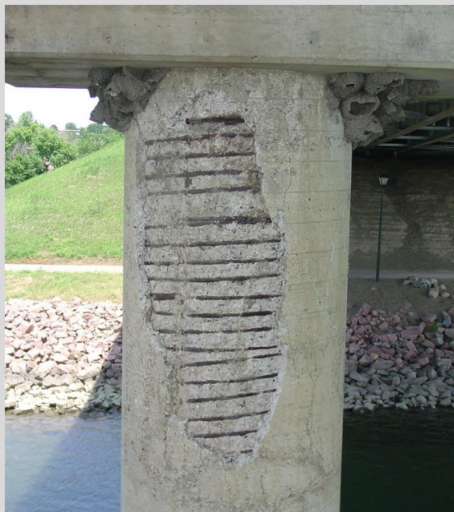
Condition State 3 Spalling (exposed and corroded reinforcement) near the top of a reinforced concrete column.
