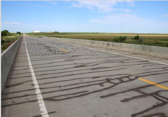
Condition State 2 Sealed cracks (medium width) on a reinforced concrete bridge deck
