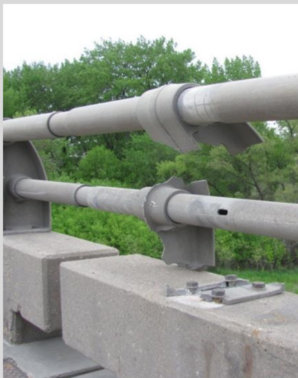
Condition State 4 Aluminum rail post severely damaged
