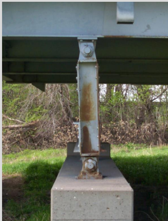
Condition State 2 Paint failure and surface corrosion on a pinned steel column
