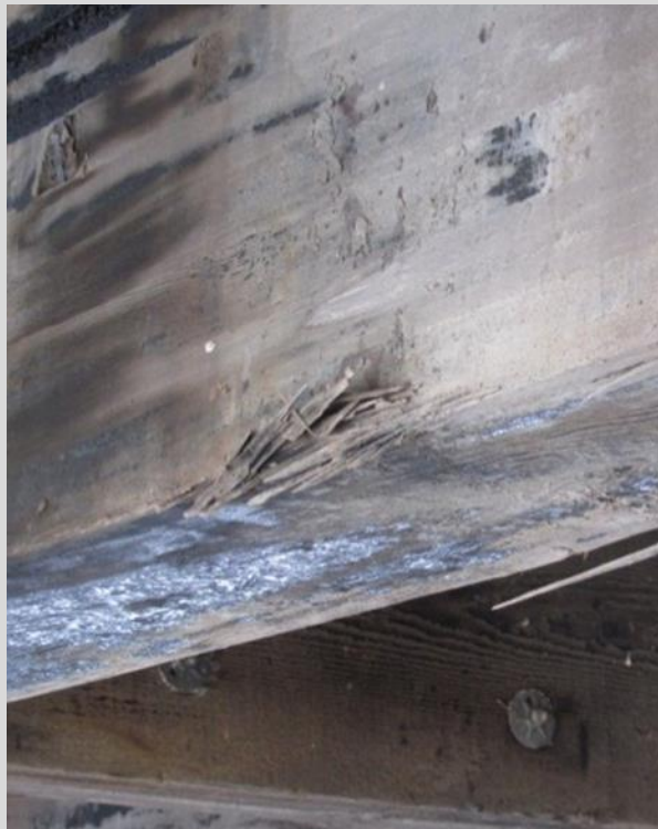
Condition State 2 Minor impact damage on a glulam timber beam.
