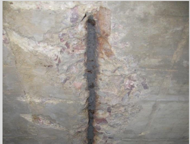
Condition State 3 Spalling (exposed rebar) on a cast-in-place (CIP) concrete box culvert.
