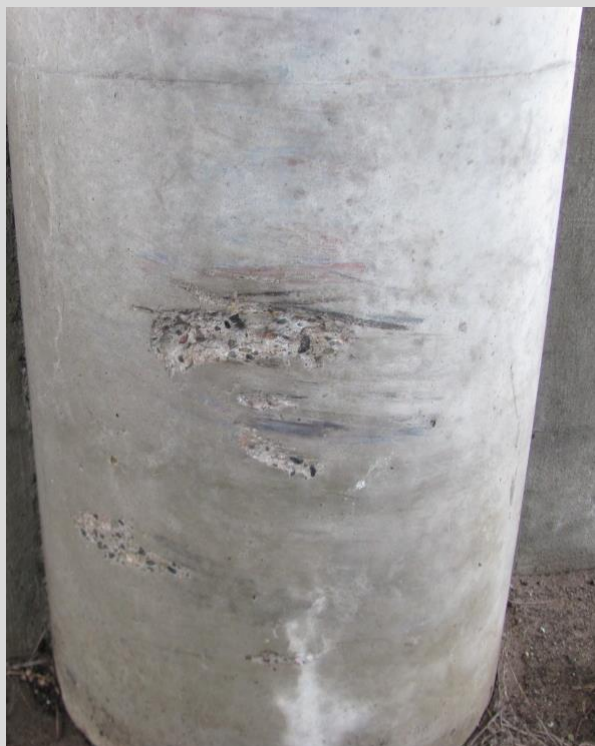
Condition State 2 Isolated impact spall on a reinforced concrete column.
