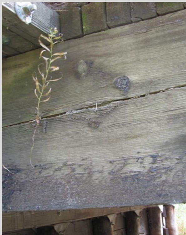
Condition State 3 Horizontal splitting with internal decay (plant growth) on a sawn timber beam.
