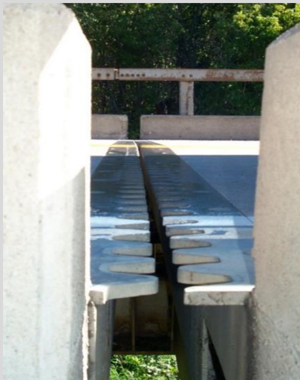
Condition State 4 Finger joint is opened beyond design limits (gap between the two finger plates)
