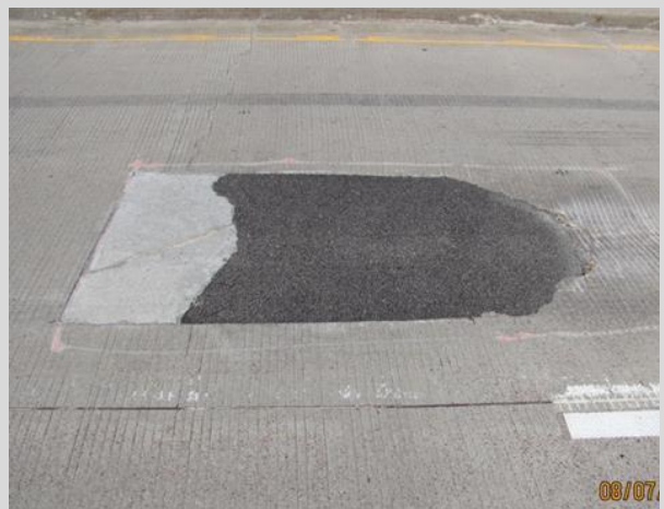
Condition State 3 Bituminous patch on a low slump concrete overlay
