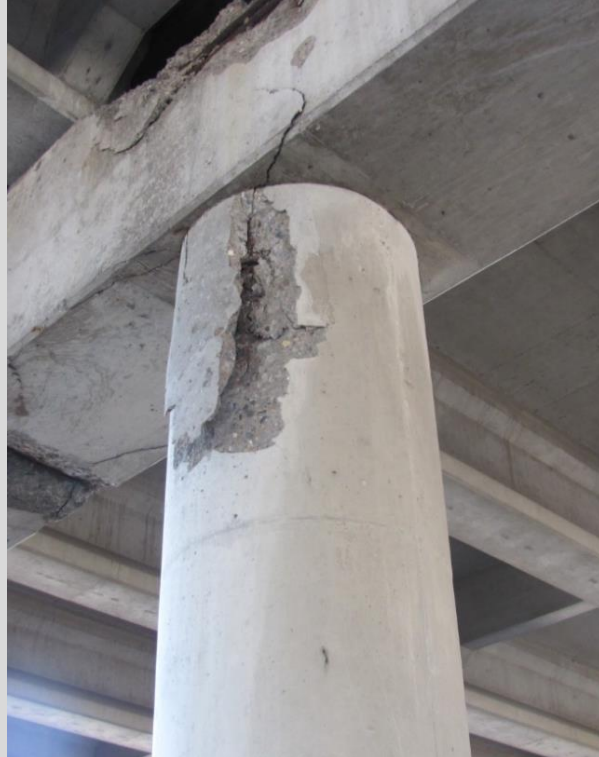
Condition State 4 Severe spall on a reinforced concrete column.
