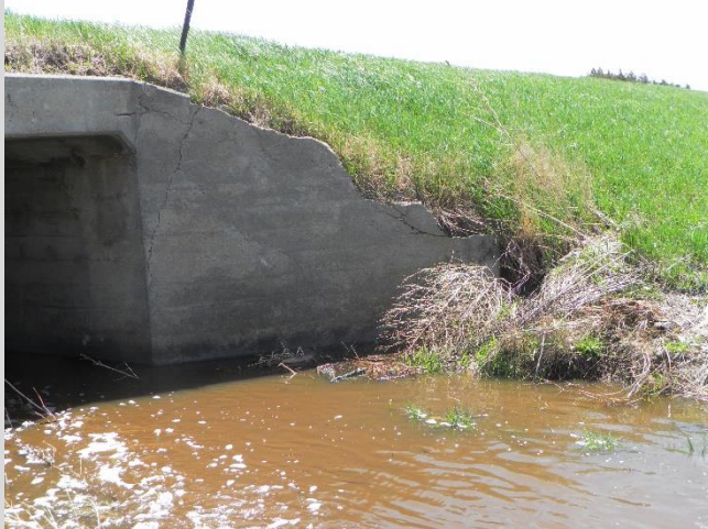
Condition State 4 Severe spalling and deterioration along the top of the wingwall.
