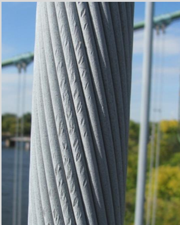
Condition State 2 Minor wear on steel strand hanger cable.
