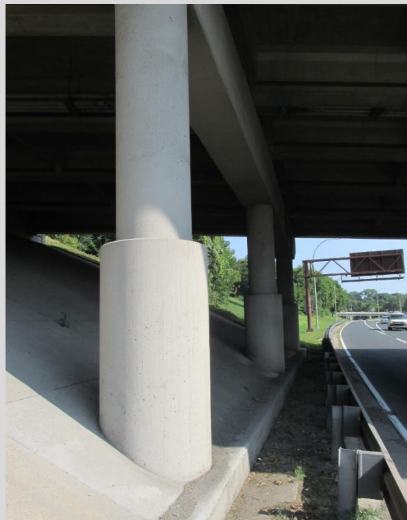
Condition State 2 Repair on a reinforced concrete column.
