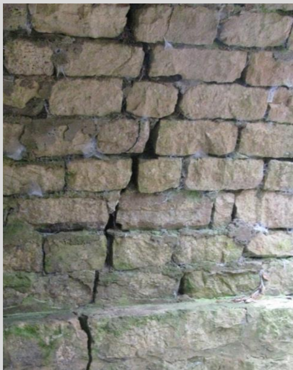
Condition State 4 Severe vertical fracture (with blocks misaligned and loose) on a masonry arch culvert.
