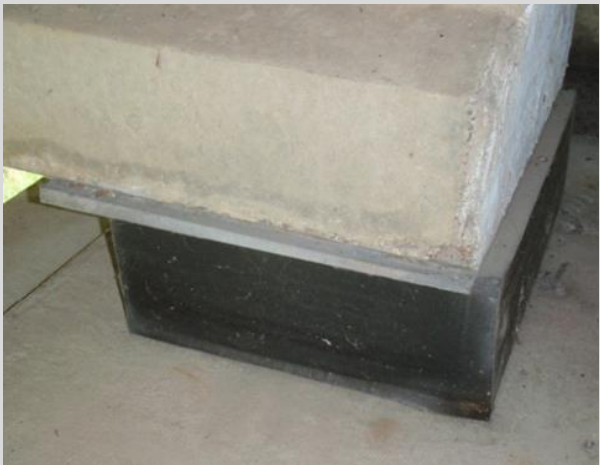
Condition State 2 Pad rolled up slightly on the bottom edge and moved from beneath sole plate (less than 1/2").
