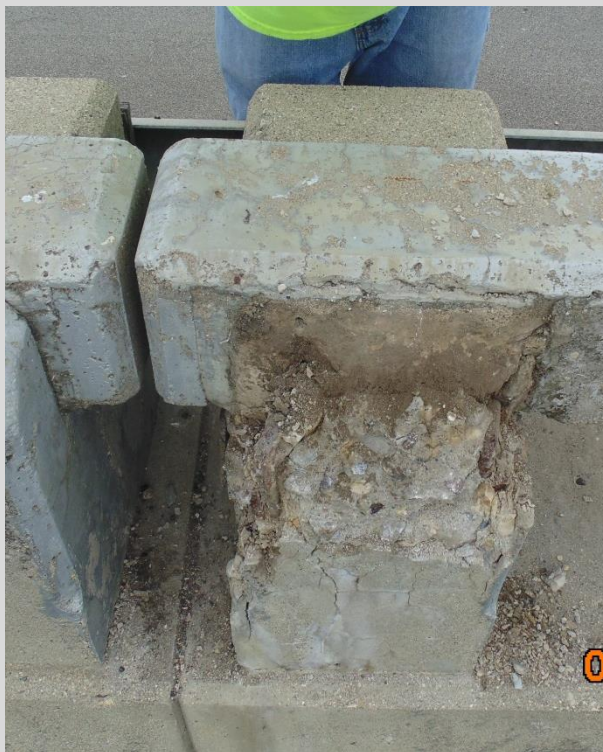
Condition State 4 Severe spall and fracture on a concrete post
