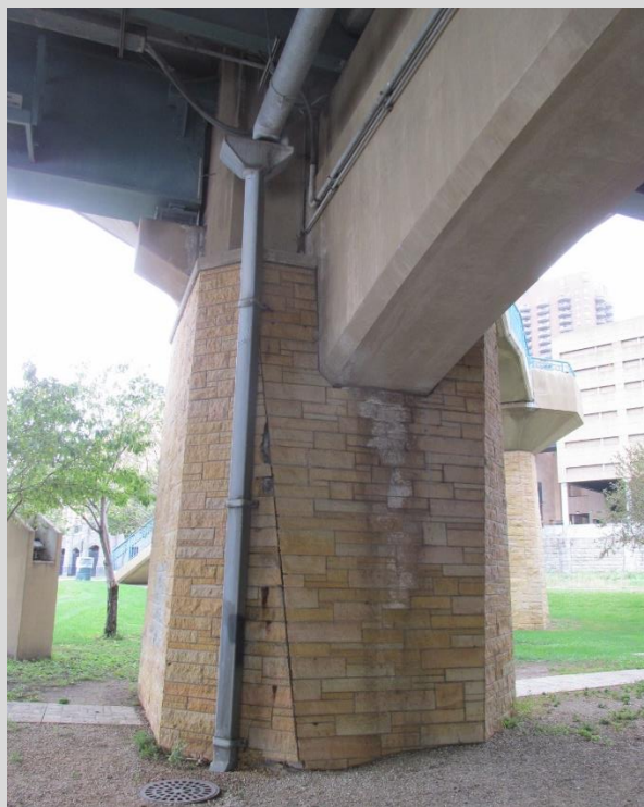
Condition State 2 Isolated loose and missing stone veneer.
