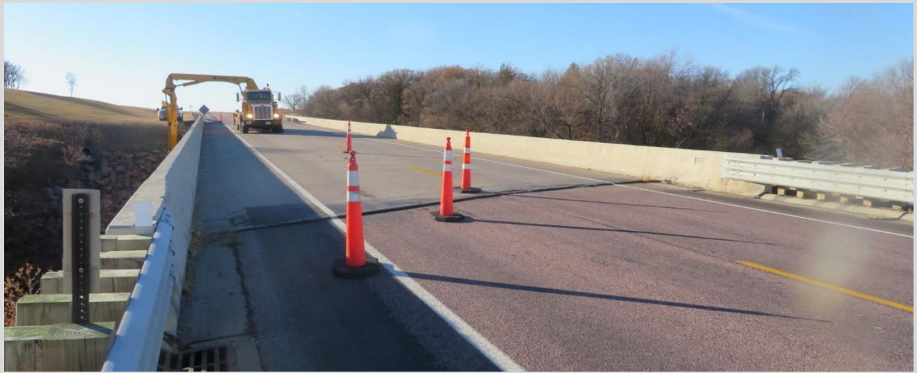
Condition State 3 (Asphalt Approach) Significant truck movement noted at the end of the bridge.
