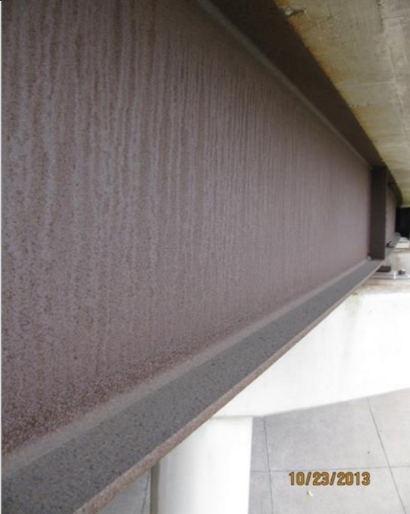
Condition State 1 Weathering steel patina is uniform and tightly adhered to the steel beam.
