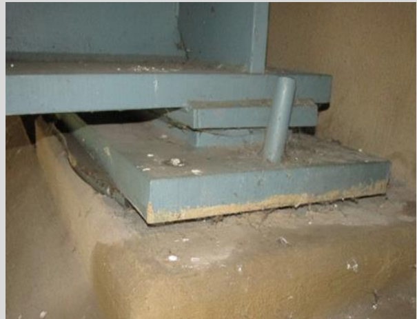
Condition State 2 Elastomeric pad is extruding and anchor bolt projects 4" above bearing.
