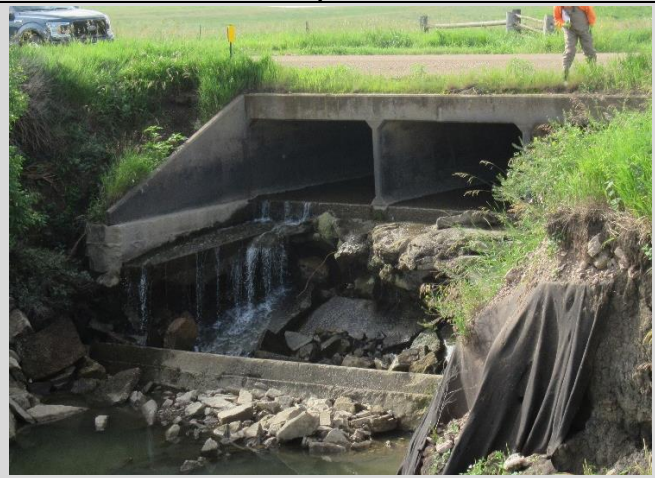
Condition State 4 Failure of the apron and the cutoff wall.
