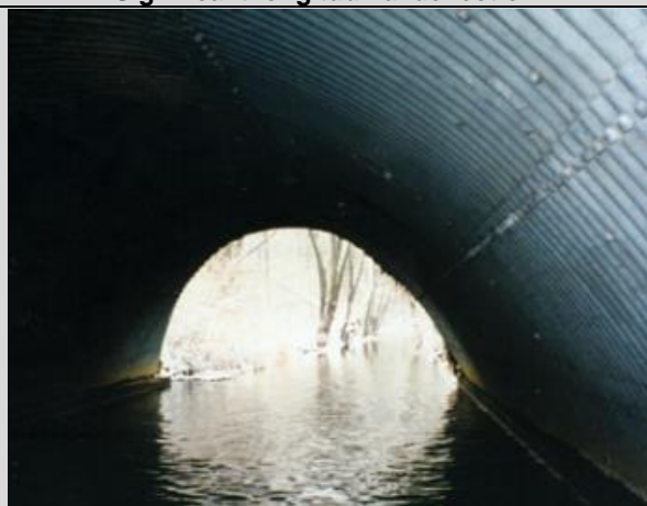
Condition State 3 Asymmetrical barrel distortion.
