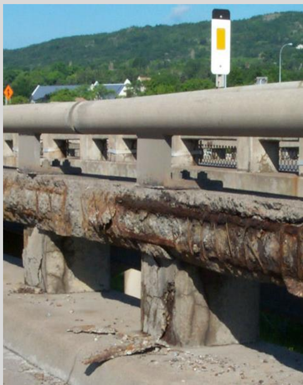
Condition State 4 Severe spalling on the concrete rail base of a combination railing
