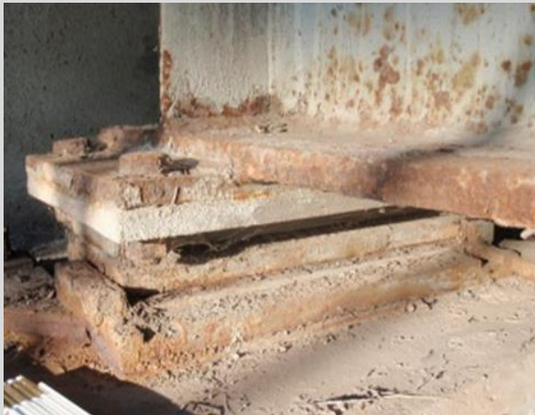
Condition State 2 Debris and surface corrosion on sliding plate bearing.
