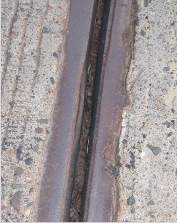
Condition State 2 Strip seal gland partially pulled out
