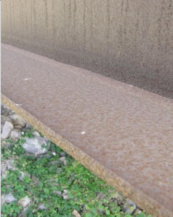
Condition State 2 Weathering steel patina is slightly uneven – surface is granular and dusty.
