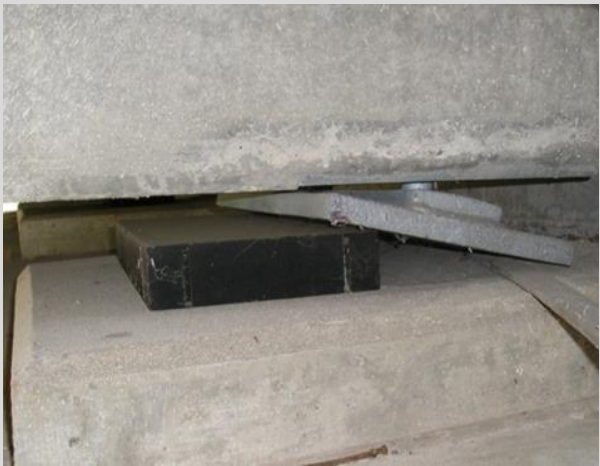
Condition State 4 Pad has moved from beneath the curved pintle plate (nearly fallen off).
