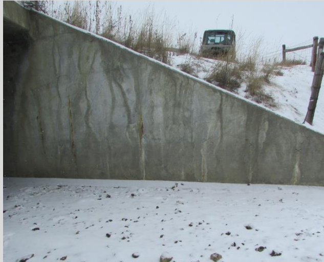
Condition State 2 Moderate cracking and light leaching along the front face of the wingwall.
