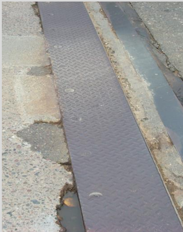
Condition State 3 Spalling and temporary patching along a sliding plate deck joint (does not impact joint function)
