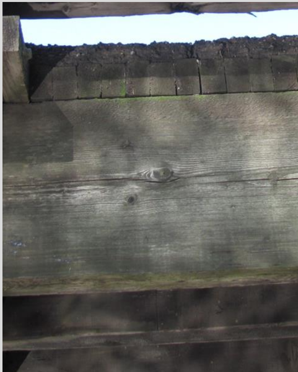
Condition State 2 Moderate horizontal splitting on a sawn timber beam.
