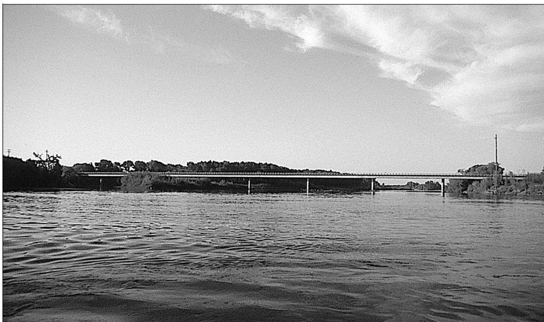
Figure 14.A-B — BRIDGE VIEW (Looking Upstream)
