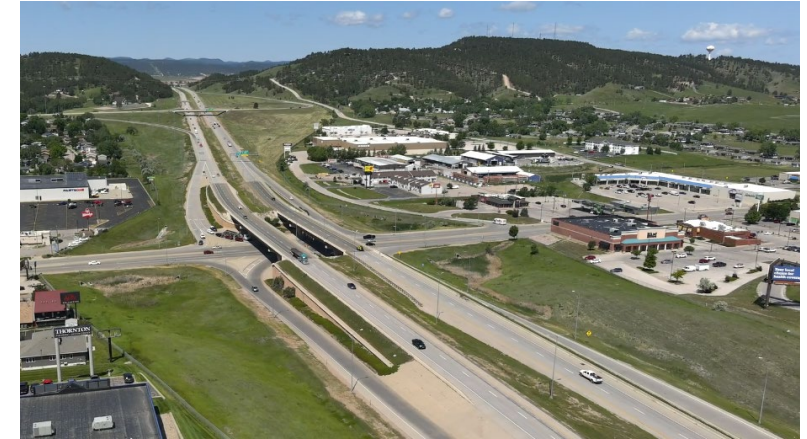
I-90 at Exit 58 (Haines Avenue) looking west.
