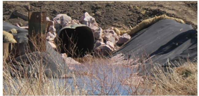
Stream diversion on a Turner County project. Culverts with a 60-inch diameter were used to divert the creek around the project area. (SDDOT)
