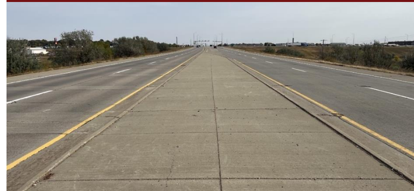
Example of a four-lane roadway with Raised Median West of Marion Road
