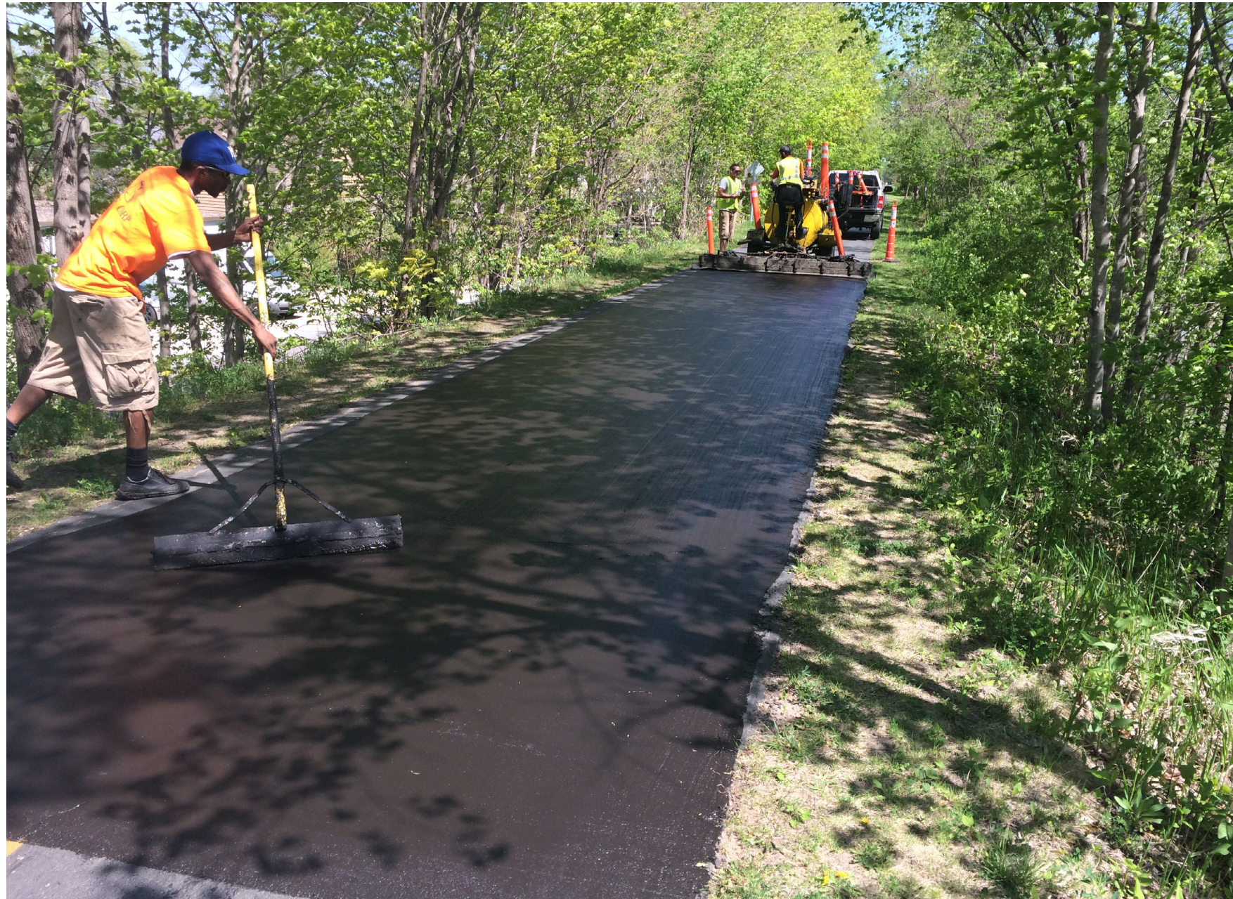
Crack/fog sealing or microsurfacing asphalt trails to extend life span.
