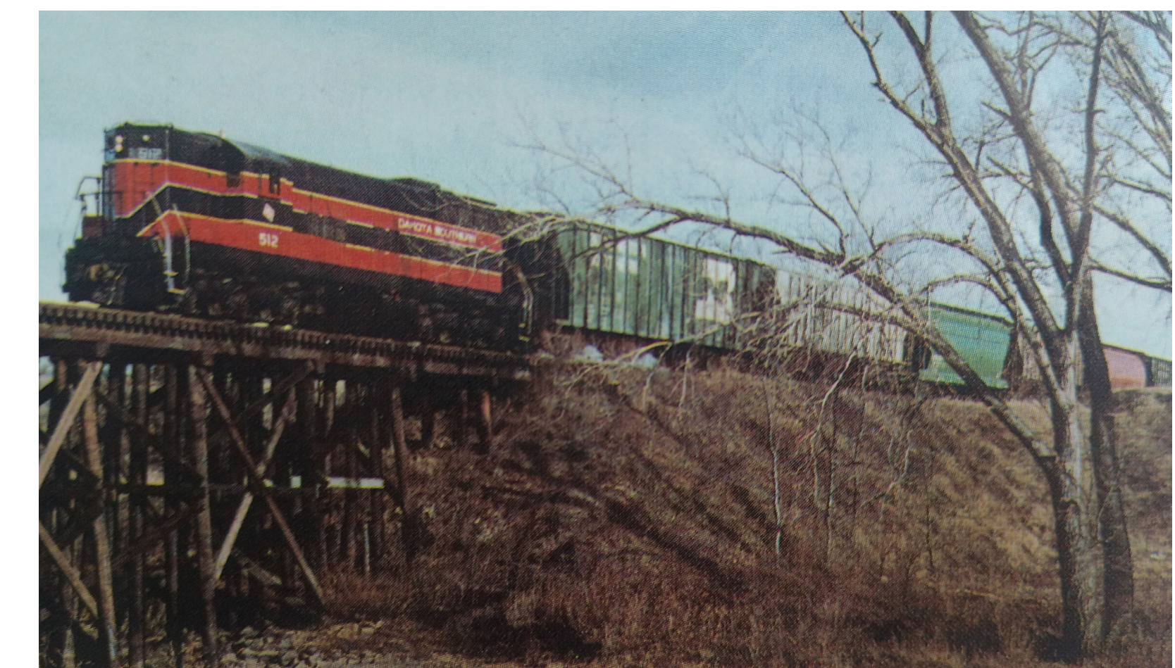
A train crosses the Emanuel Creek trestle west of Tyndall in December 1988. Credit: Rick VanZee
