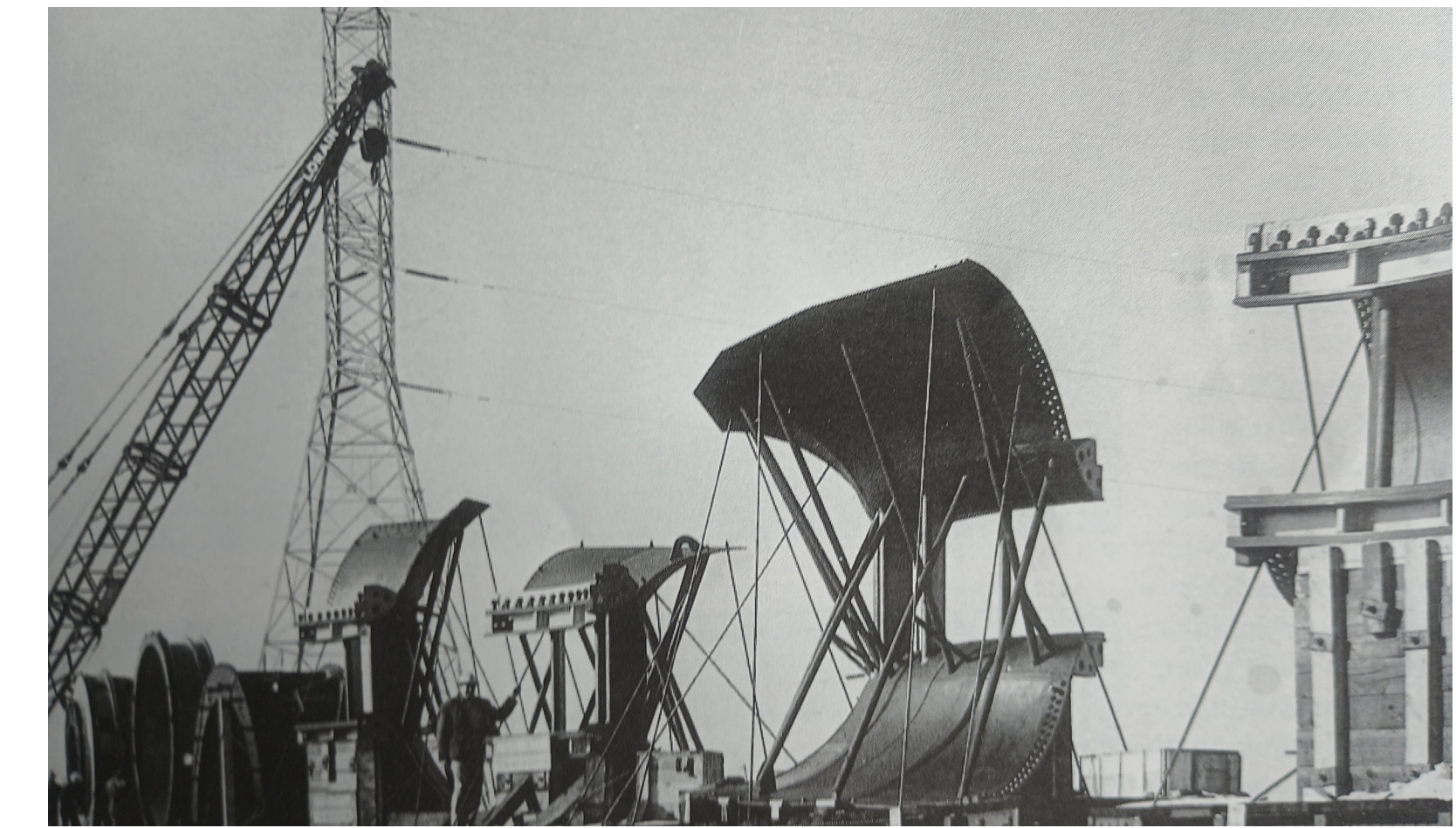
Steel for Fort Randall Dam on railcars is unloaded in 1953, after traveling along the Platte line. Credit: U.S. Army Corps of Engineers
