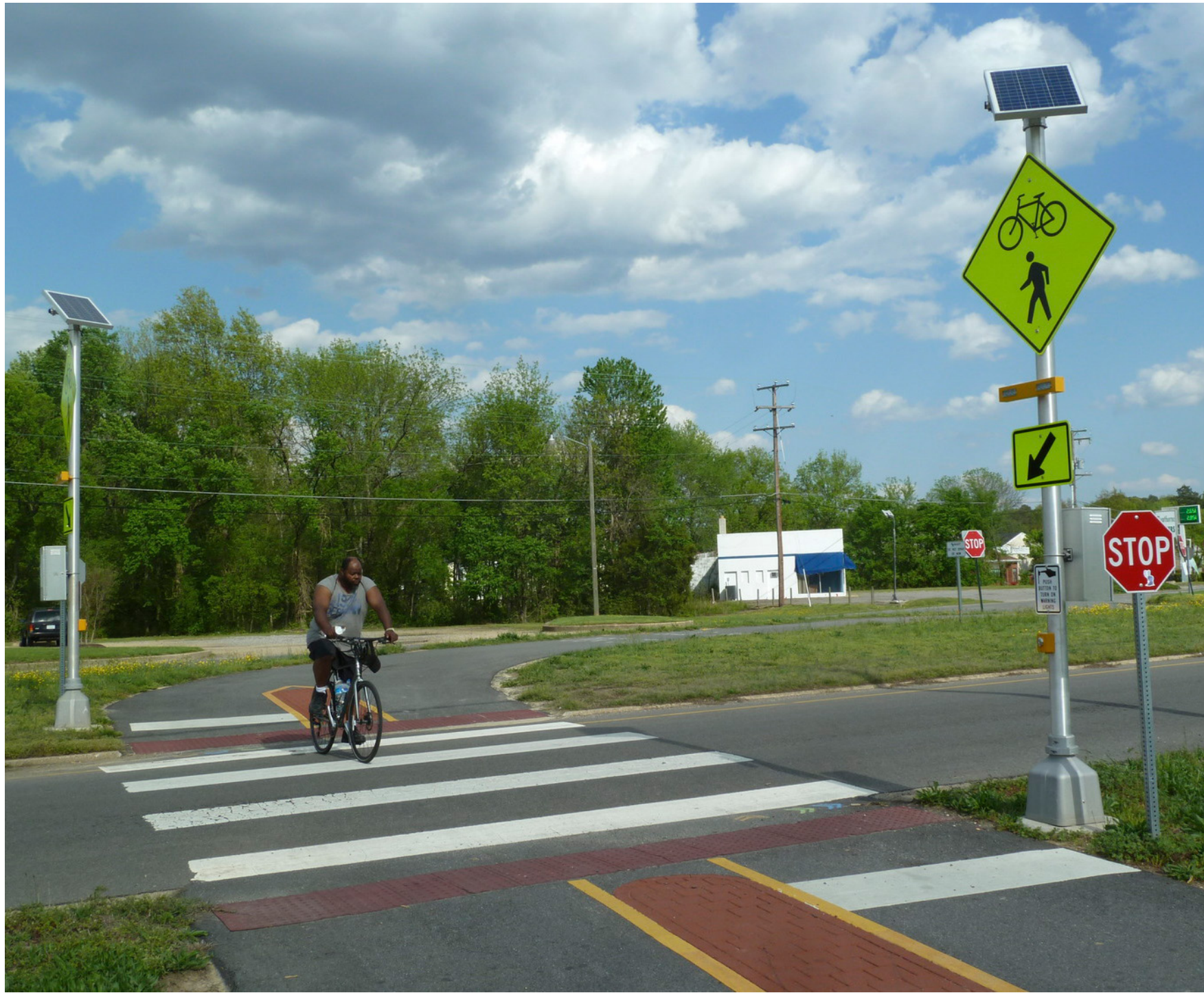
Maintaining pavement markings and signs at road crossings.
