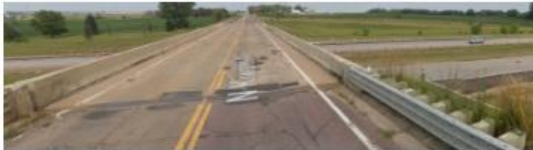
Photo of Kiwanis Bridge Deck Showing Approach Repairs
