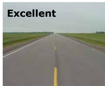
Excellent Smooth pavement with no rutting and no cracking
