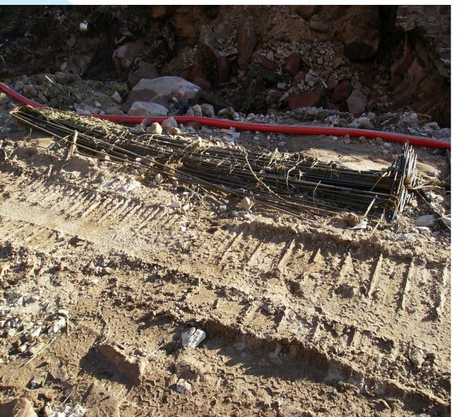
Do not stockpile where equipment could damage the steel rebar
