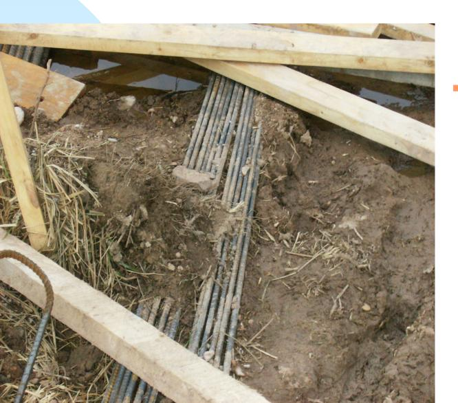
Do not drag on ground to prevent damage to the reinforcing steel or contamination of the steel rebar
