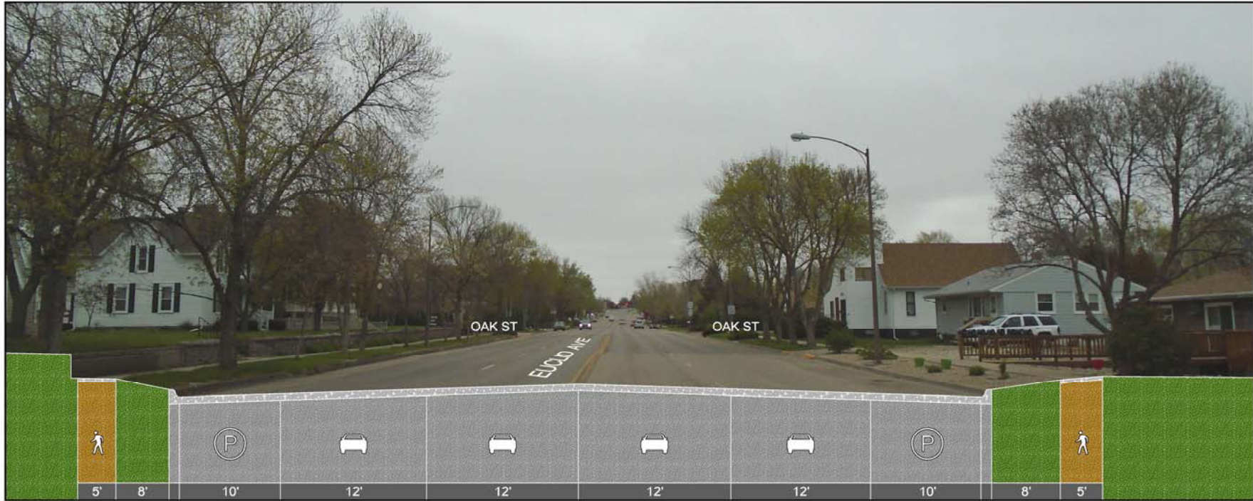
EXISTING 4-LANE SECTION - 68' LOOKING NORTHBOUND AT EUCLID AVENUE & OAK STREET
