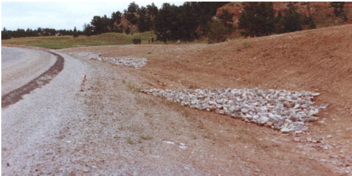
Figure 5.20 Rock Check Dams
