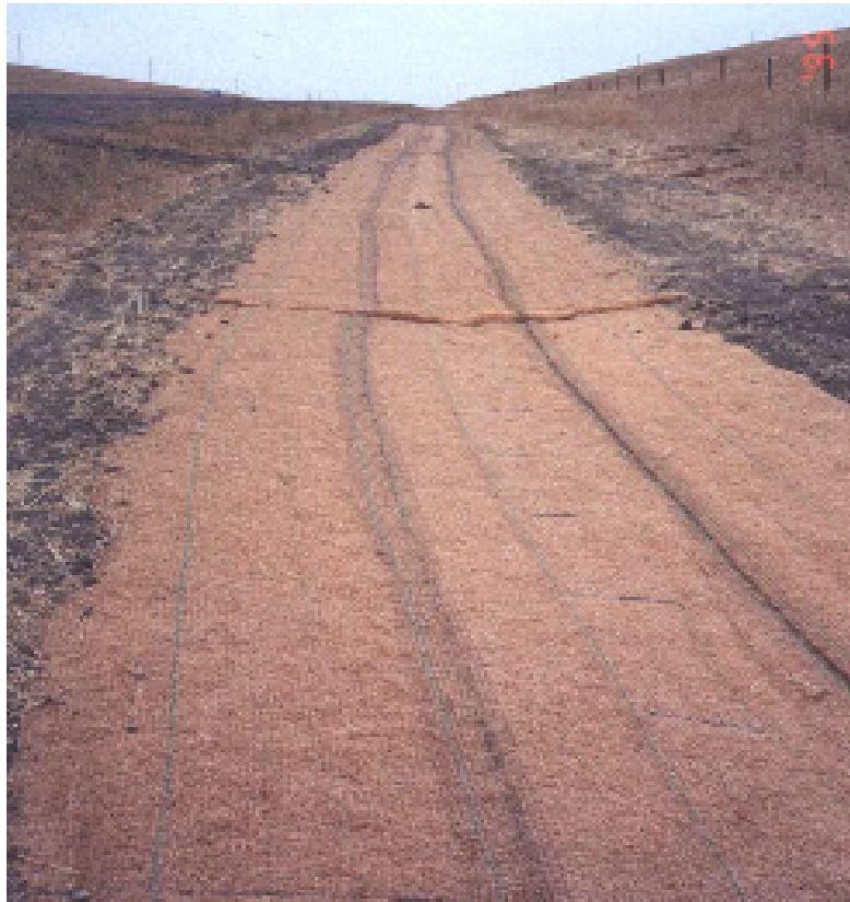
Figure 5.9 Properly Installed Blanket
