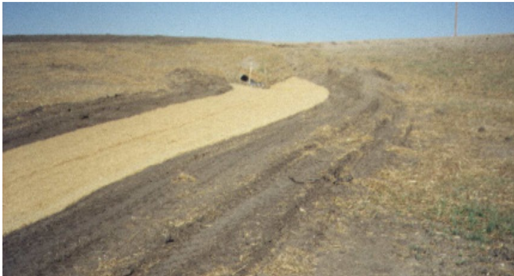
Figure 5.3 A Properly Prepared Channel
