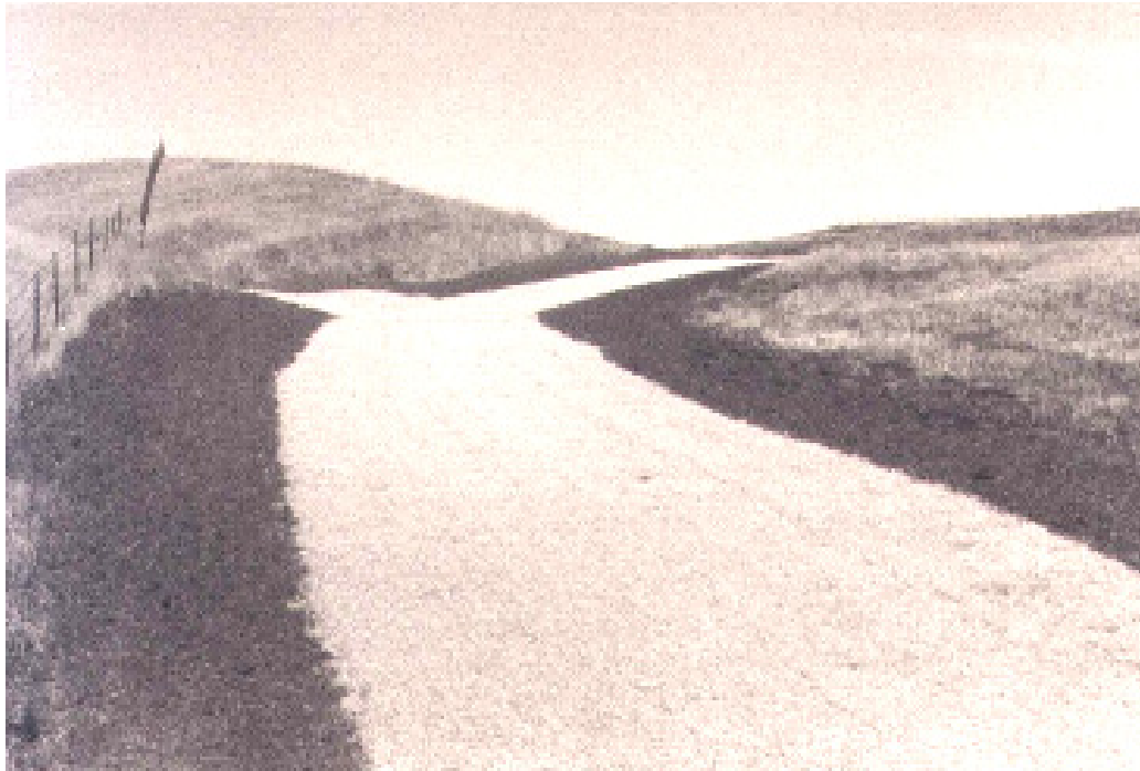
Figure 5.4 A Properly Shaped Channel
