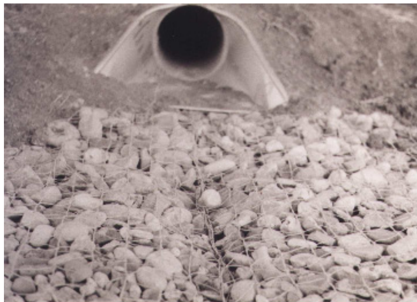
Figure 5.26 Gabions used at Pipe Outlet
