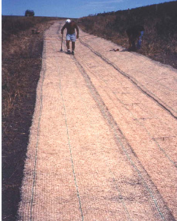
Figure 5.6 Properly Installed Erosion Control Blanket
