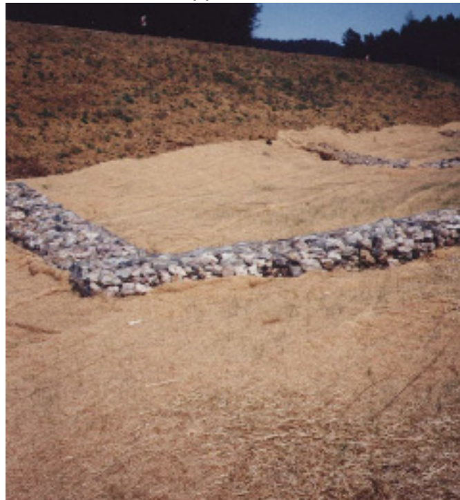
Figure 5.25 Gabions used in a Channel Application.
