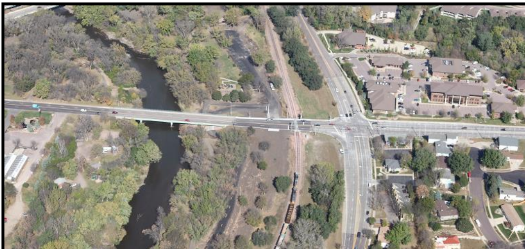
Existing 26th Street Big Sioux River Bridge that would remain as part of the No-Build Alternative.
