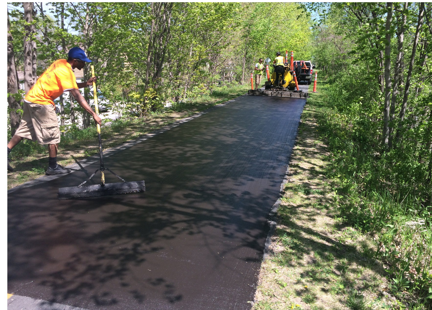
Crack/fog sealing or microsurfacing asphalt trails to extend life span.
