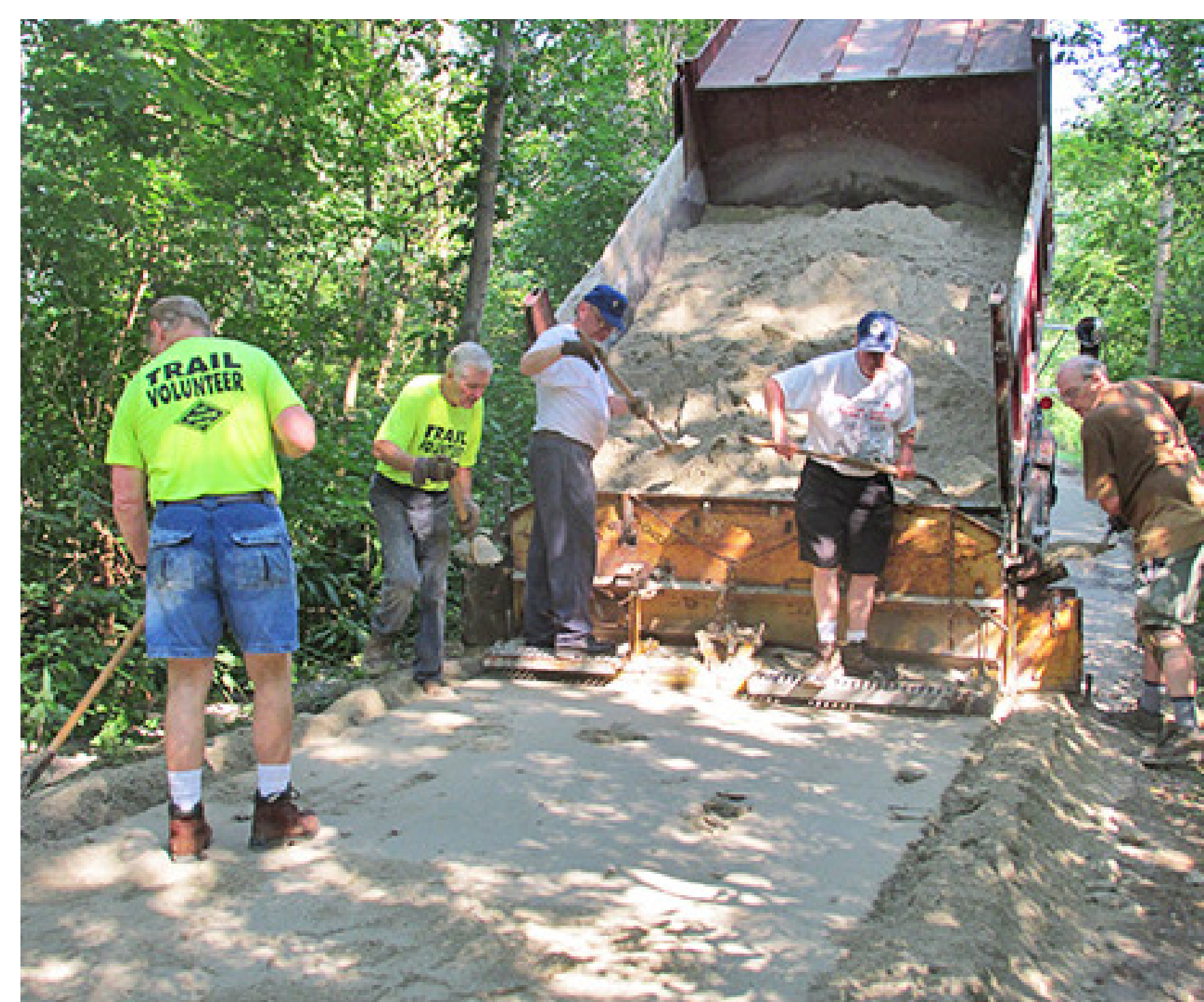
Adding and compacting crushed stone. Credit: Montour Trail Council
