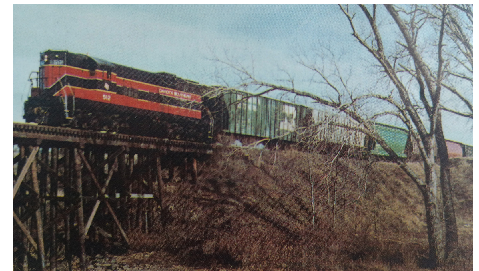
A train crosses the Emanuel Creek trestle west of Tyndall in December 1988. Credit: Rick VanZee
