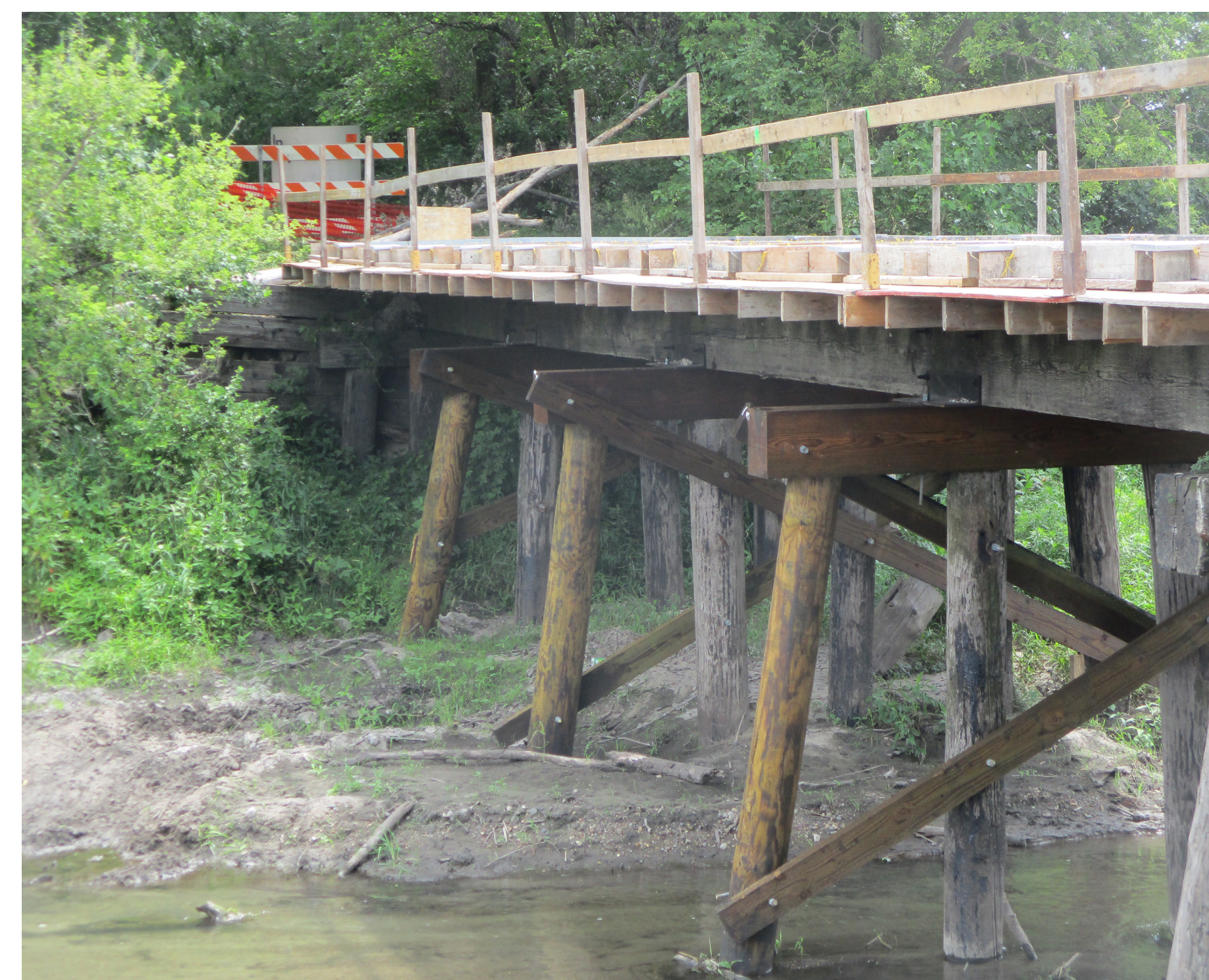
A former railroad bridge undergoing repair and conversion for trail use.
