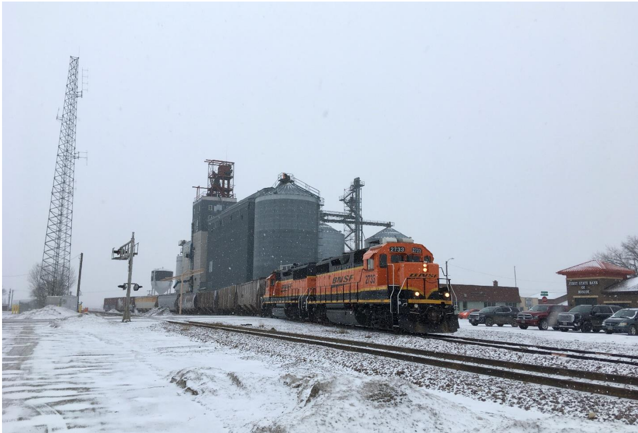
Figure 4: BNSF Railway Serving Grain Elevator at Roscoe, South Dakota
