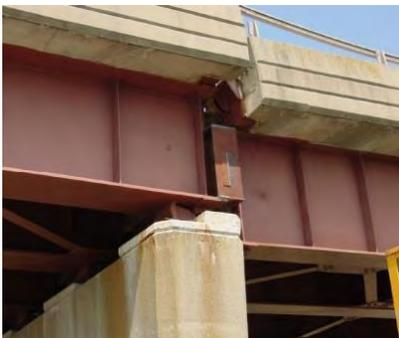
The 2005 collapse of the Dunn Bridge in Albany, New York was attributed to the malfunction of the rocker bearings, combined with horizontal deflection of the supporting pier. The rocker bearings had been misaligned for several years prior to the collapse.
