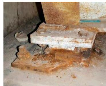
Corroded (possibly frozen) sliding plate bearing
