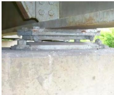
**Uplift (gap) on a curved plate fixed bearing**
