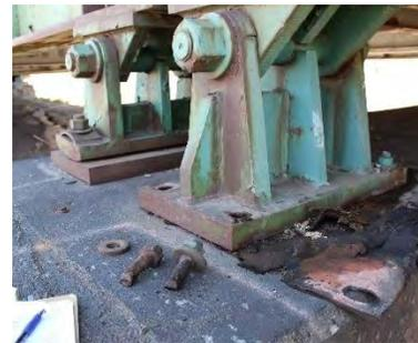
**Anchor bolt failure on a fixed bearing**
