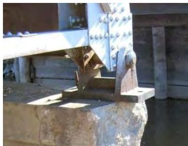
Fixed pin truss bearing with severe loss of bearing area
