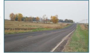
Typical McCook County highway cross-section with bituminous surfacing.
