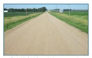
Typical McCook County highway cross-section with gravel surfacing.
