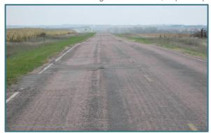
The 1-mile segment of 448th Avenue (CH 5), between Lake County and 245th Street, is a candidate location for bituminous to gravel surface conversion. Low traffic volumes, deteriorating pavement condition, and a gravel-surfaced roadway in Lake County are all considerations.
