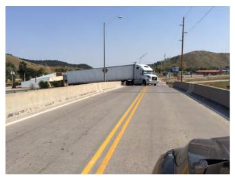
In addition, the skew of the interchange creates conflicts between vehicles on the bridge and semi-tractor trailer turning movements at the ramp terminal/service road intersections, as depicted in the photo on the left (photo credit: A. Olson, September 2015).
