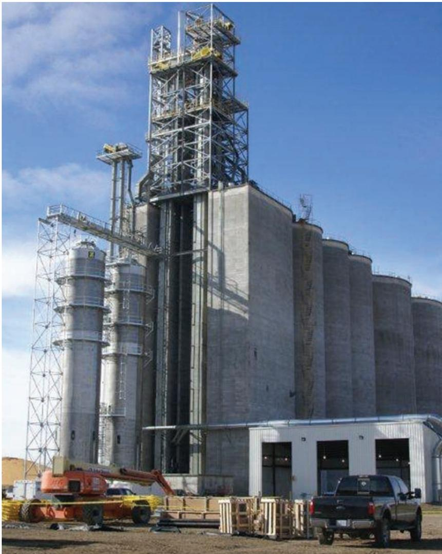
*The Gavilon Liberty Grain LLC high-speed grain and dry fertilizer shuttle facility includes a 2.2-million-bushel, upright concrete grain elevator, a 42,000-ton dry fertilizer facility and a 1.5-mile loop track large enough to accommodate 125 cars.*
