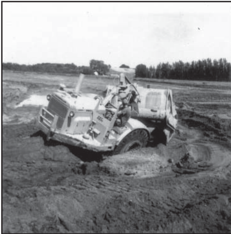
Earth Mover, Interstate Construction, 1960, 84-088, 5277B
