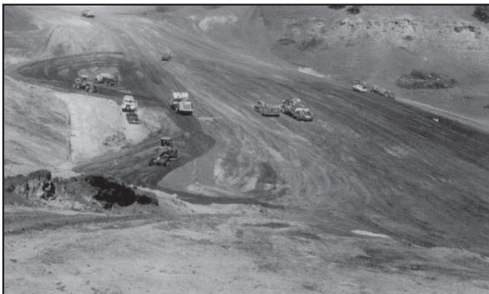
Interstate Construction, making a path up hill, 84-088, 5277B
