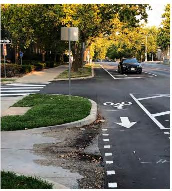
Buffered bike lane with buffer separating bicycles and on-street parking. This arrangement uses parked cars to provide additional separation. (Armour Boulevard, Kansas City, MO)
