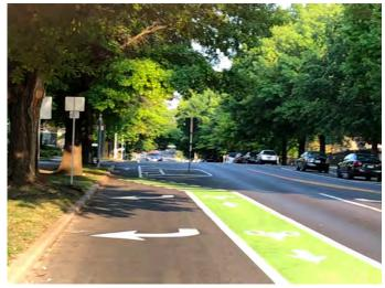
Green paint is used to mark conflict zones as motor vehicles cross the bike and and buffer to make right turns.
