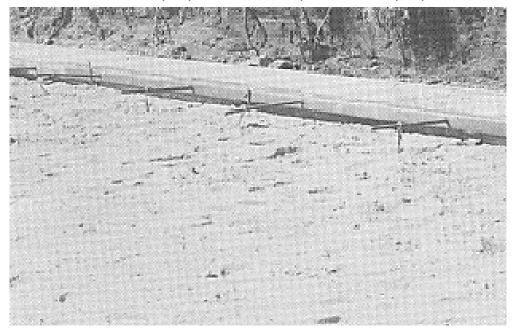
Figure 3.28 Keyway strip in slab.
