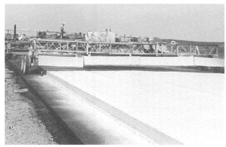
Inspect the coverage. If any areas do not have uniform coverage, adjust the equipment and respray.
