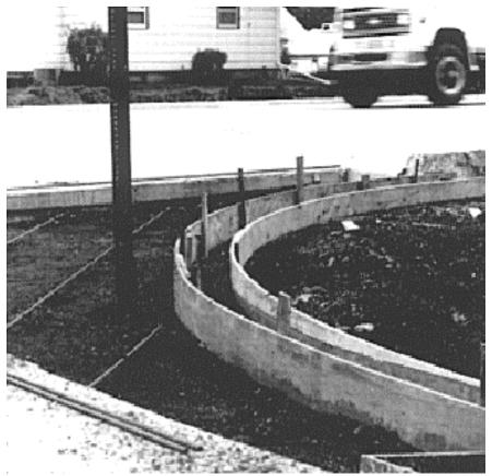
Figure 8.2 Slip-form paving curb and gutter.
