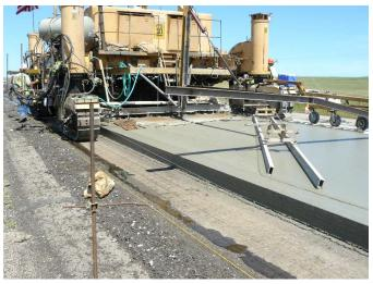
Electronic sensors follow a fixed stringline, which is used for elevation control, and must guide the forward movement of the slipform paver.
