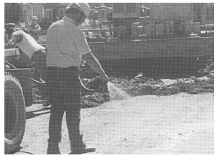
Figure 5.12 Spraying water on finegrade.
