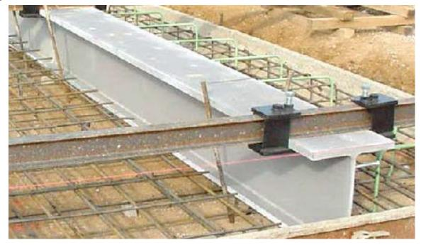
Figure 4.15 Pavement terminal beam
