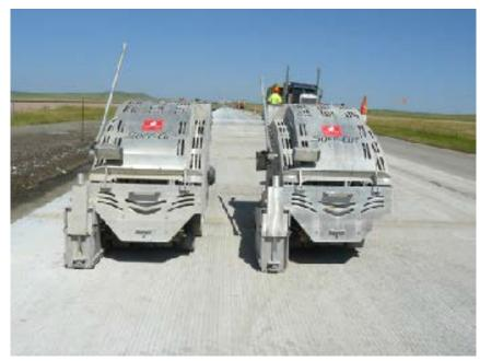
Figure 7.5 Concrete saw.
