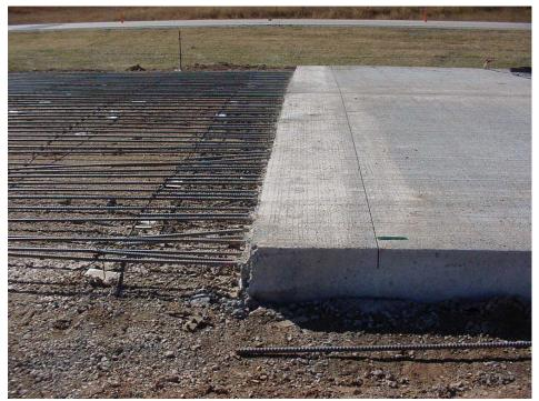
Extra care is needed to ensure both concrete quality and extra consolidation at these joints. The inspector must ensure that the header is placed correctly. A straight edge should be used to determine correct placement of the header. The inspector should assure that there is adequate vibration around reinforcing bars through the construction joint and vibrate a sufficient distance back from the construction joint to assure that all the concrete has been properly consolidated.
