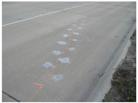
Stitching of a longitudinal uncontrolled crack is needed when the centerline tie bars were not placed or placed improperly during construction.
