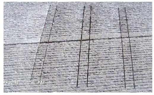
Figure 9.7 Dowel bar retrofit installation
