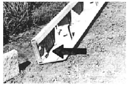
Figure 3.5 A curve having a radius over 100 feet formed by using 10-foot straight sections.
