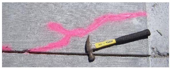
Repair or correction of uncontrolled cracks (**380.3 L 4**) shall be as directed by the Engineer and at the expense of the Contractor.
