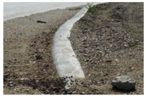
Figure 3.10 Poorly set top of transverse header form.
