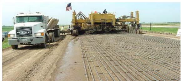
Figure 4.1 Placement of continuously reinforced concrete pavement (CRCP)
