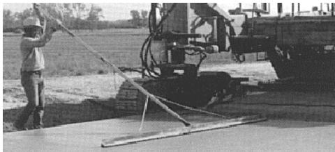
Figure 6.1 Surface check with straightedge behind the paver.
