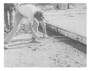
When the transverse construction joint will become the contraction joint location, the correct size dowels must be used to ensure load transfer. The dowels must be centered over the new working joint location and placed parallel to the surface and perpendicular to the centerline. Dowel baskets are commonly modified or cut apart for this type of header.
