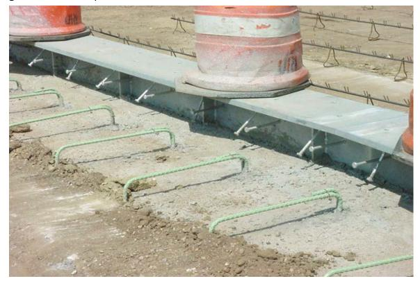
Figure 4.17 Close-up of concrete anchors on the nonreinforced side.
