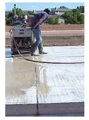
Figure 7.3 Joints are sawed into concrete after it has hardened.
