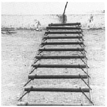
Dowel bars shall be placed parallel to the subgrade and parallel to the centerline of the pavement. Misaligned dowels either vertically or horizontally are a cause of joint failures. Always check the Standard Plates in the plans for dowel bar tolerances.
