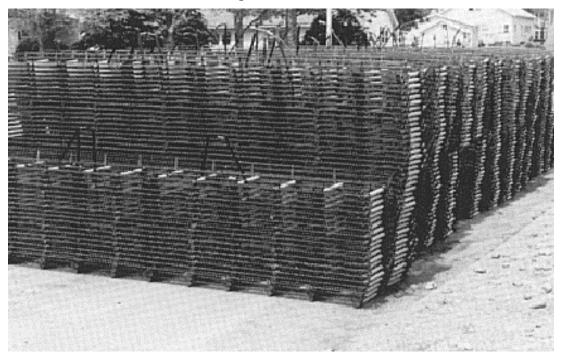
Do not allow dirt or grass covered dowel baskets to be placed. These create voids around the bars. Future joint failures might occur. If dowel baskets are to be stored on site for more than 30 days, cover them as per **480 3 A**.
