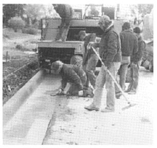
The basic requirements (base preparation, form setting, stringlines, finishing, etc.) for either of the two curb and gutter construction methods are similar to those for mainline paving. However, transitions in the curb and gutter for radius and fillets at intersections, approaches for driveways, etc., require handwork.
