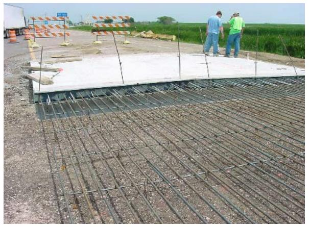
The inspector should also be watching the reinforcing steel during the concrete placement by either the spreader or paver. The plastic concrete being pushed ahead of either the spreader or paver puts a large amount of pressure against the reinforcing steel and can cause misplacement of the reinforcing steel. Experience has shown that tieing the steel to far ahead of the paver causes the reinforcing steel to bend due to the pressure from the paving operation.
