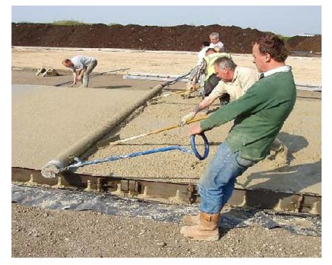
**Figure 5.24** Picture of a Truss Screed which is used for small formed placements. These screeds normally have cable and a winch that moves the screed forward.
