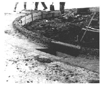
Figure 8.3 Fixed form curb and gutter prior to hand finishing.
