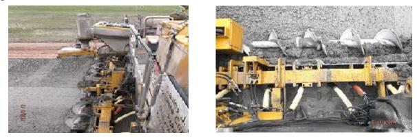
Consolidation throughout the pavement slab is important, including the form line when stationary form paving. If the paver vibrators do not affect the edges of the slab, a hand operated internal (spud) vibrator should be used to eliminate honeycombing. Internal vibrators used <u>next to forms</u> shall have a frequency of not less than 3500 impulses per minute. **(380.3 B 5)**
