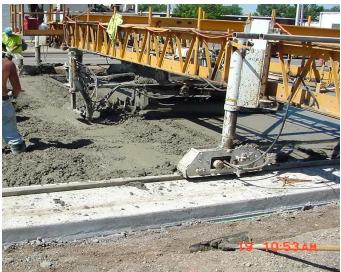
**STRINGLINE SLIP-FORM PAVING (SLIPFORM PAVING)** is the construction method used to spread and finish concrete in one operation, eliminating the need for forms. This method is commonly used on major PCC paving projects.
