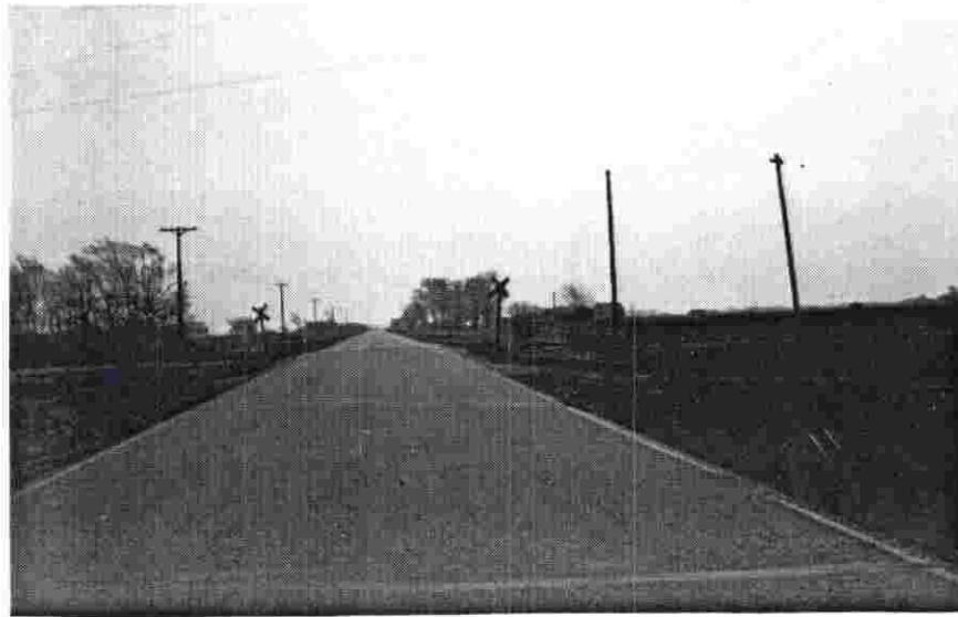
FAIRGROUNDS ROAD - Eastbound
