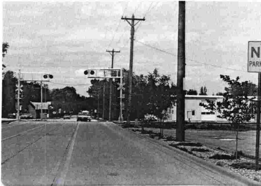
DAKOTA STREET (MAIN LINE) - Northbound
