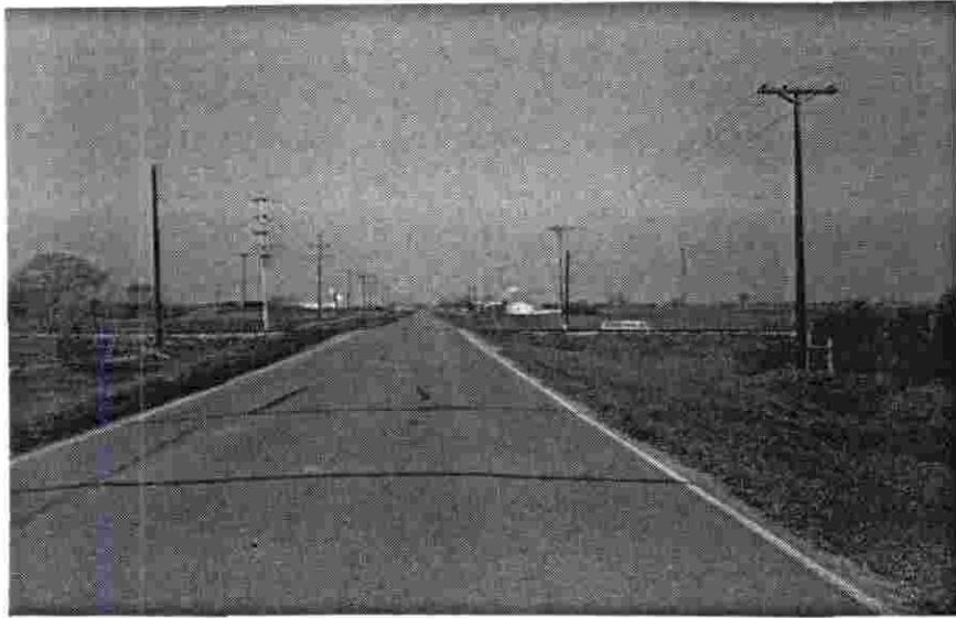
FAIRGROUNDS ROAD - Westbound
