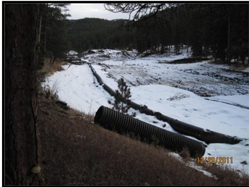
Figure 3. Bypass Pipe in Place for Dredging at Dalton Lake in 2011-2012
