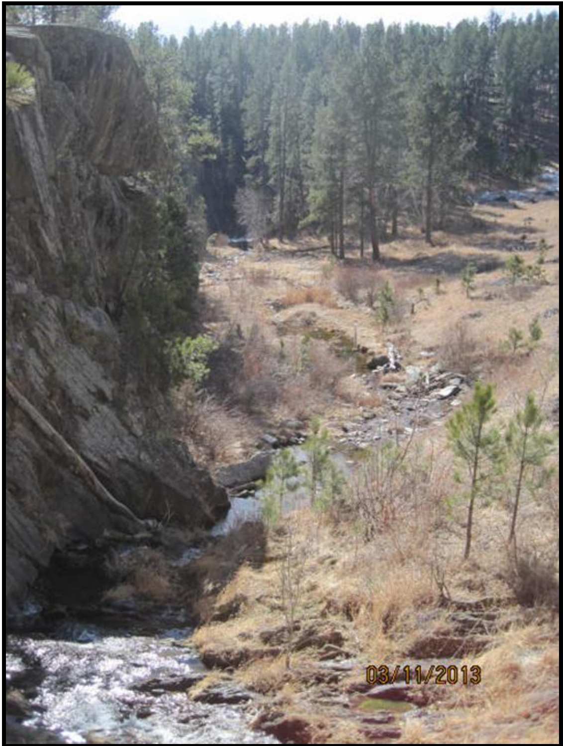
Lakota Lake outlet/spillway looking downstream.
