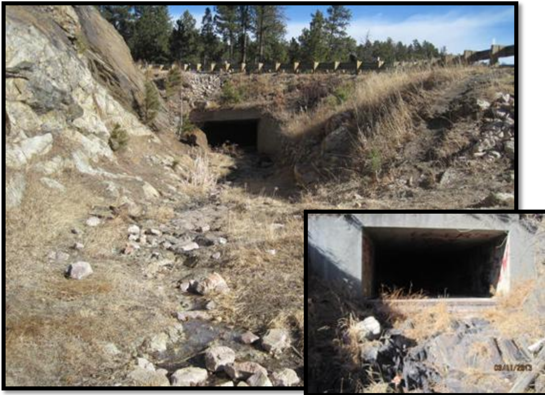
Horsethief Lake outlet looking downstream; inset photo of dry outlet culvert.
