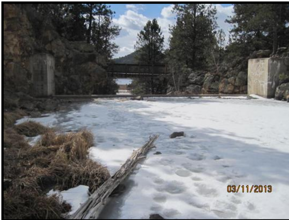
Bismarck Lake spillway with no outflow.
