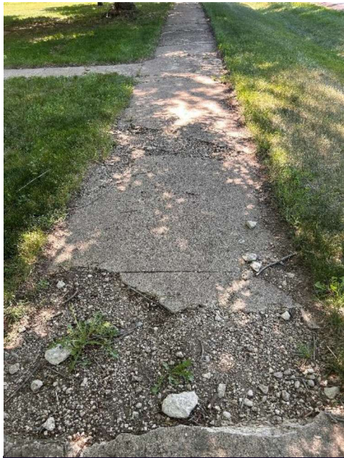
Deteriorated Panel
