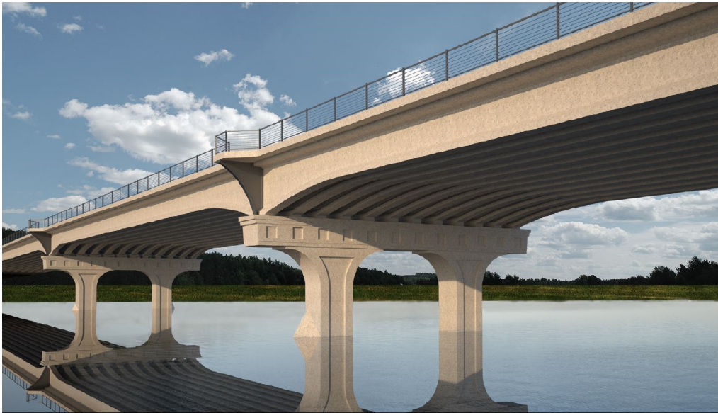
Figure 5-4: Two column pier type
