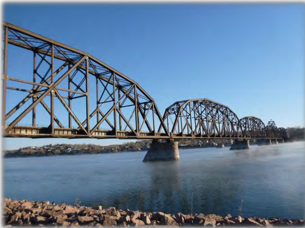
Figure 3-4: The Former DM&E Railroad Bridge
