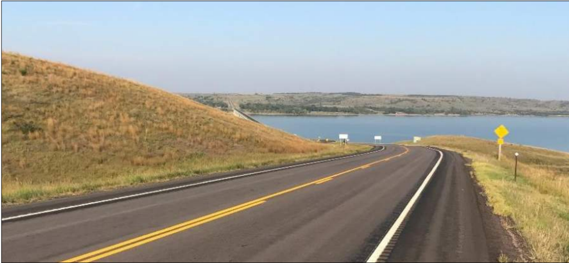
Figure 9. Visibility Concern (Eastbound SD44 Approaching the Bridge)
