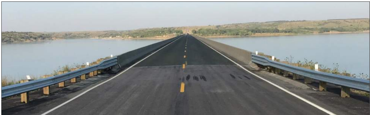
Figure 4. Existing Bridge Looking East
