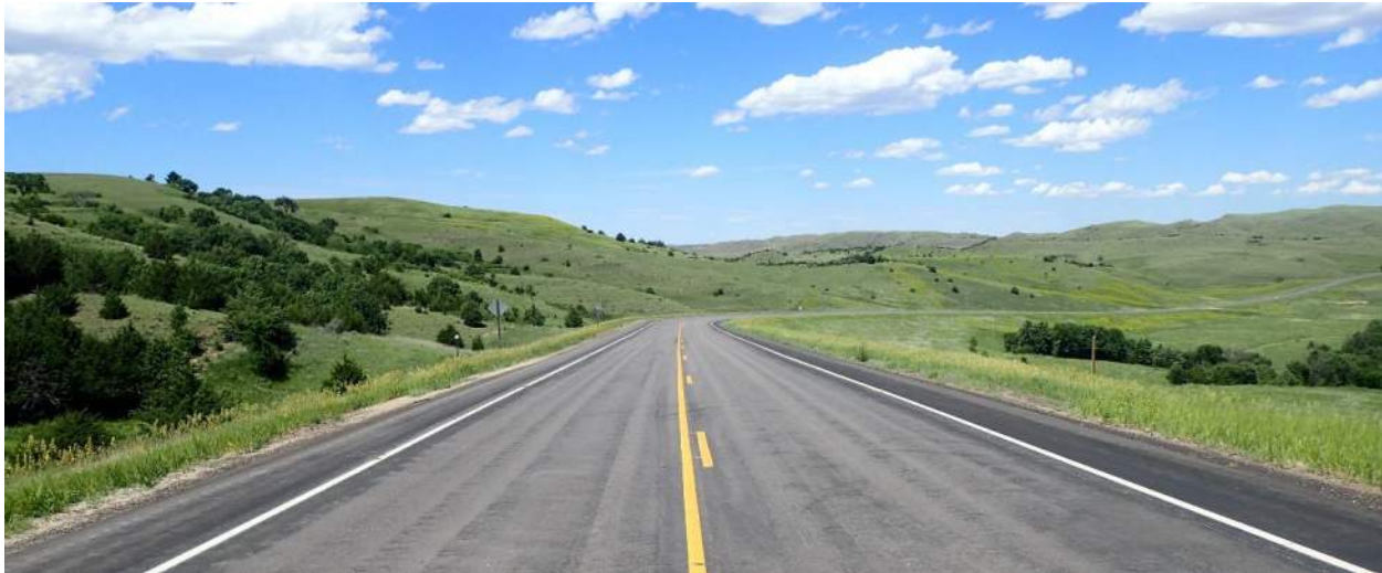
Figure 6. Existing SD44 (West of River)
