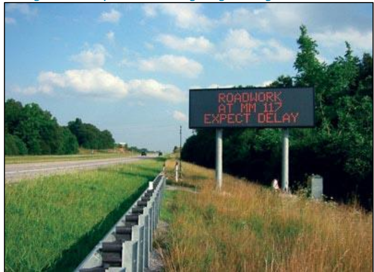
Figure IV-1: Dynamic Message Sign Along Rural Corridor
