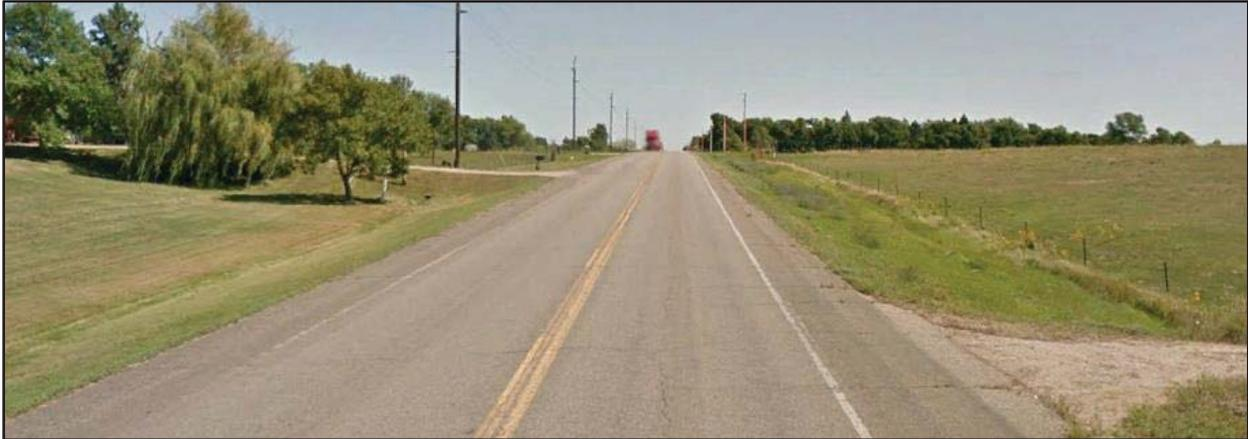
*Figure 6-18: Custer Avenue typical existing section: Narrower two-lane rural section with 1-foot shoulders*
