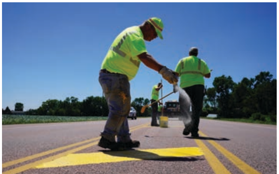
SDDOT Crews Work to Place Reflective Beads on New Pavement Markings
