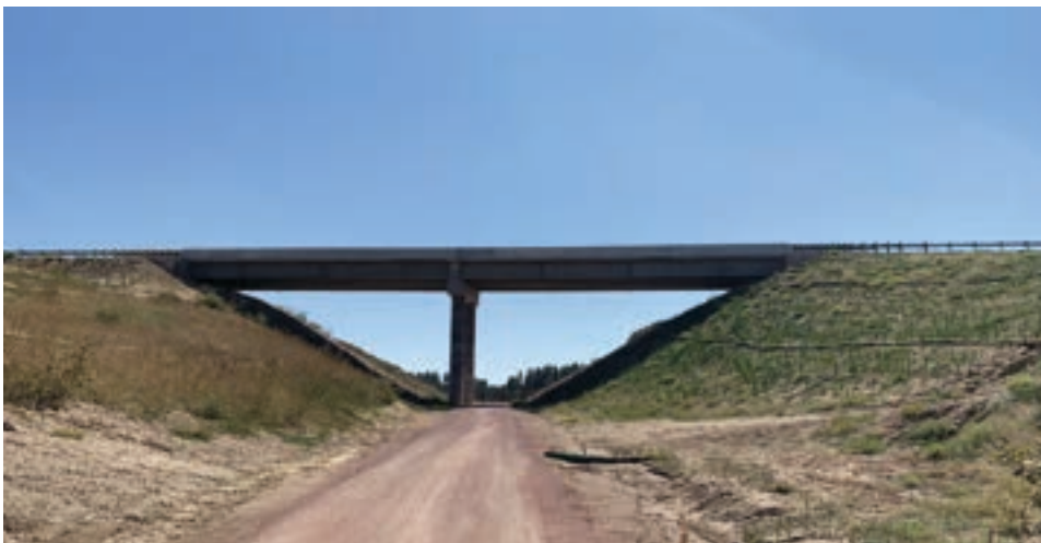
After Construction - Mickleson Trail Underneath
