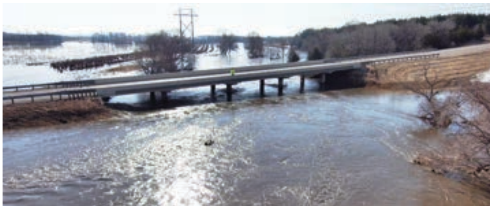
Bridge in Grant County
