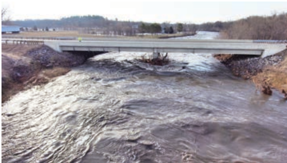
Bridge in Grant County
