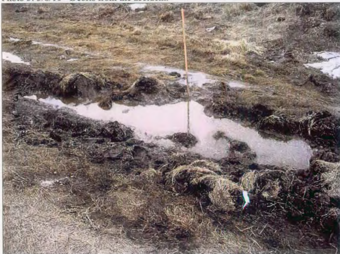
Photo 4: 3/15/10 - Pool of water after fuel was removed with adsorbent pads.
