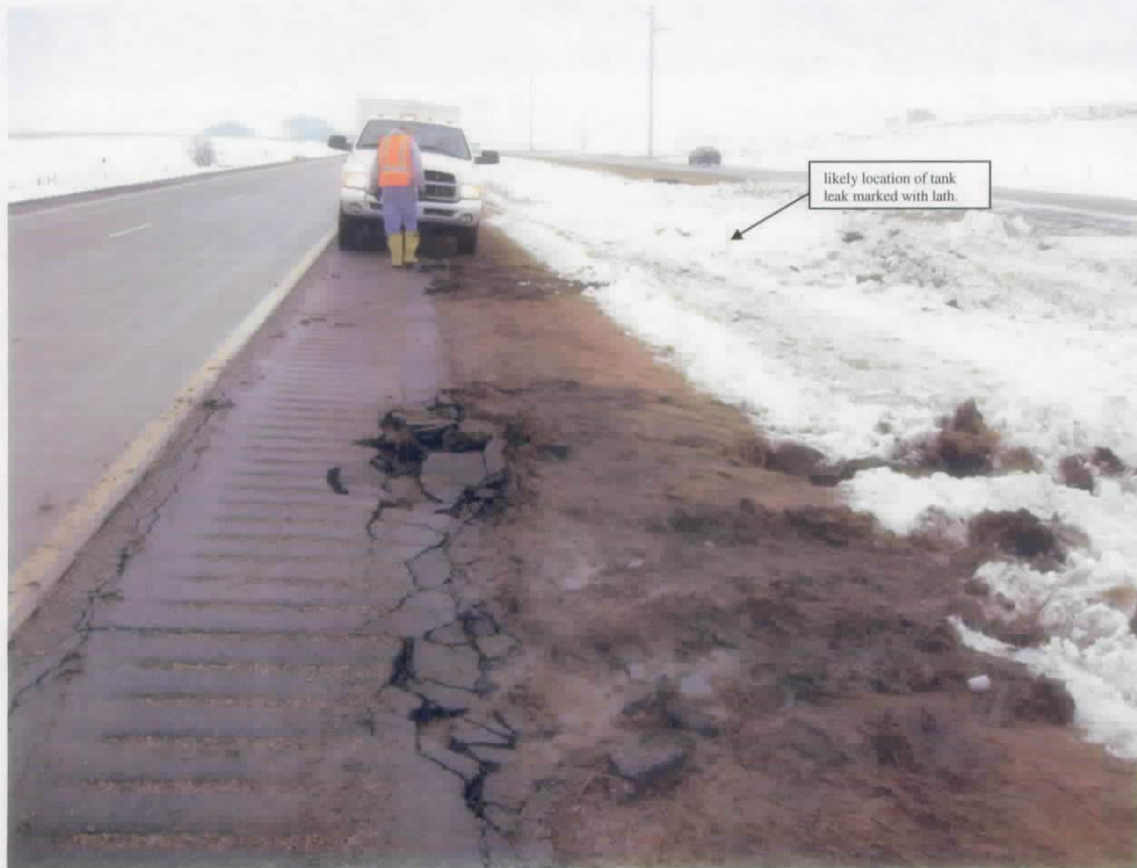
Damaged north shoulder asphalt and deep ruts in grass.
