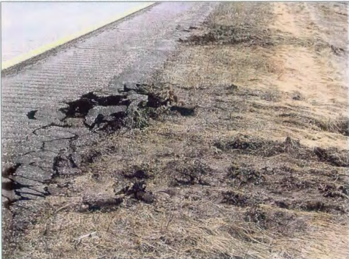
Photo 6: 3/15/10 - Damaged asphalt median shoulder.
