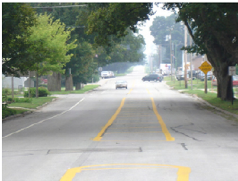
Figure 5.5. After lane narrowing was installed
