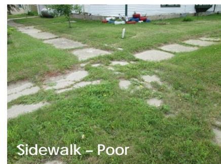
As evidenced by Figure 12, many segments of Faulkton's sidewalk system are in the "Fair" or "Poor" categories, meaning that many places, even many of those that are adjacent to a sidewalk, are inaccessible or inconvenient for pedestrians. As a result, many pedestrians have been observed walking in streets in areas where sidewalks are unavailable or in poor condition. This poses safety concerns for pedestrians and motorists alike.
