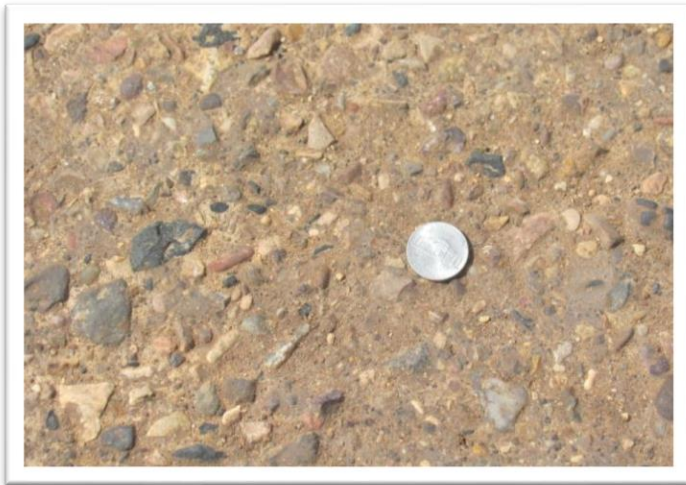
Figure 10: The above image shows a close-up view of a stabilized gravel surface as a result of chloride stabilization practices.
