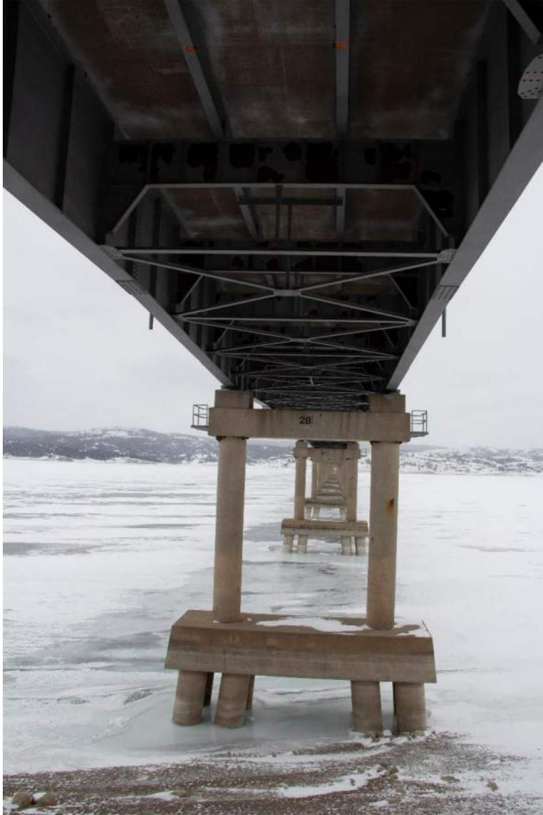
*View below easternmost spans of the Platte-Winner Bridge showing the floor system of floor beams, stringers, underside of deck, and the supporting eight-pile pier, view facing west.*
