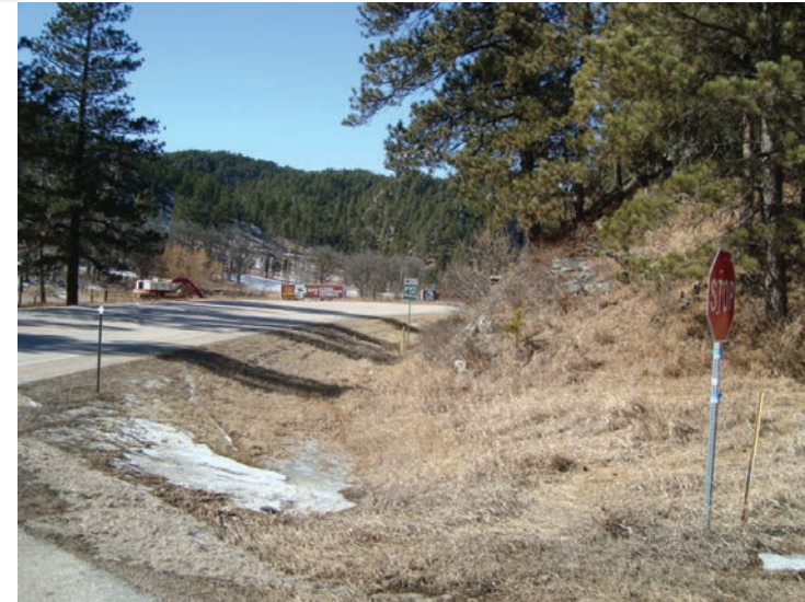
FIGURE 19 – Limited Sight Distance Facing West Along SD 40 from S Rockerville Rd
