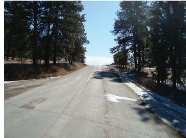
FIGURE 13 – Vertical Curvature on S Rockerville Rd (Camera Facing South)
