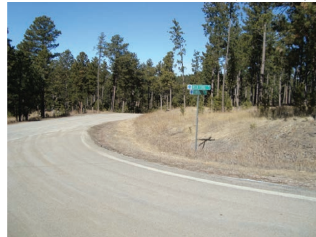
FIGURE 14 – Limited Sight Distance From Neck Yoke Road Approach (Camera Facing North Approach of S Rockerville Road)
