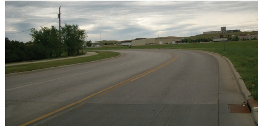
FIGURE 21 - Limited Sight Distance Facing North Along Concourse Drive
