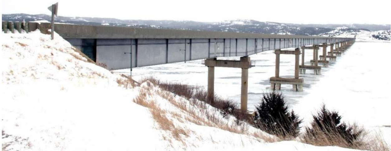
Figure 2. The Platte-Winner Bridge, view facing southwest. Mead & Hunt photograph, February 25, 2019.
