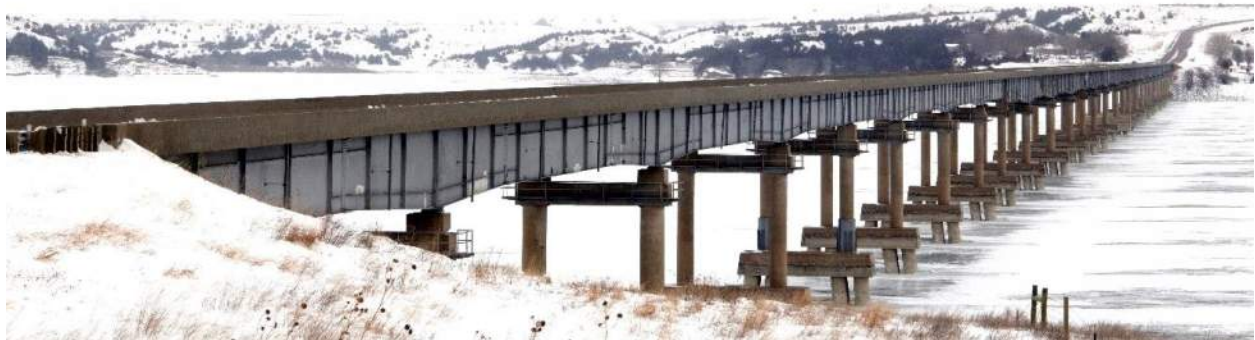
Figure 1. The Platte-Winner Bridge, view facing northeast. Mead & Hunt photograph, February 25, 2019.
