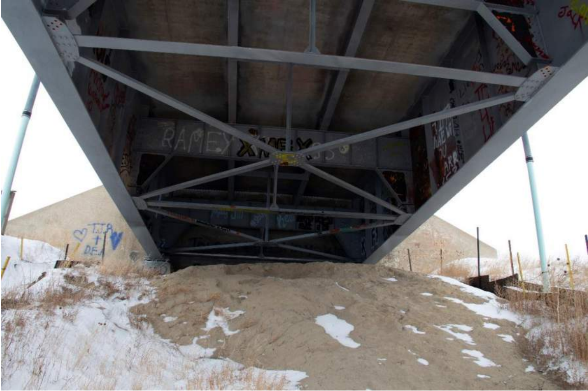
Below-bridge view of the east sill (abutment) area, view facing east.
