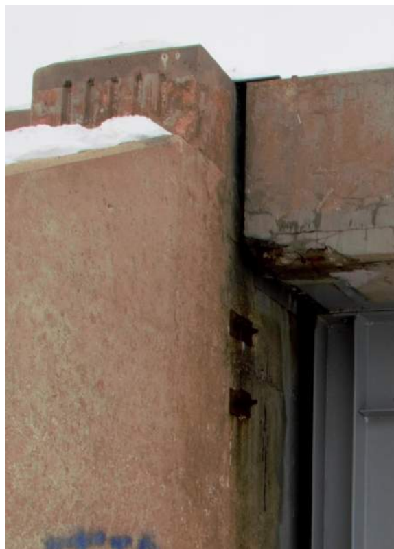
Figure 8. Endpost detail on northeast corner of the Platte-Winner Bridge, showing the set of five ornamental vertical grooves. Mead & Hunt photograph, February 25, 2019.
