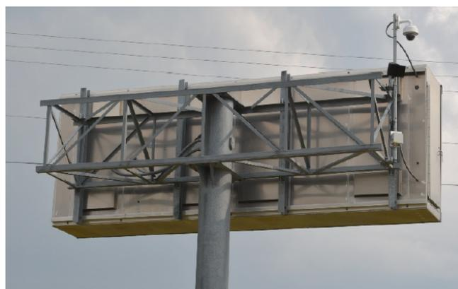
Figure 8: Closed Circuit Television
