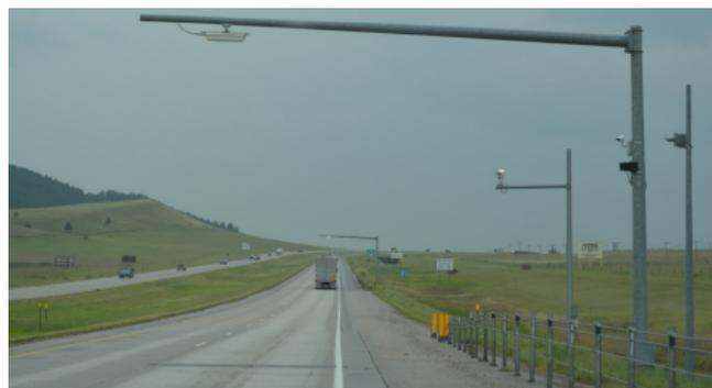
Figure 13: I-90 Weigh-in-Motion Equipment
