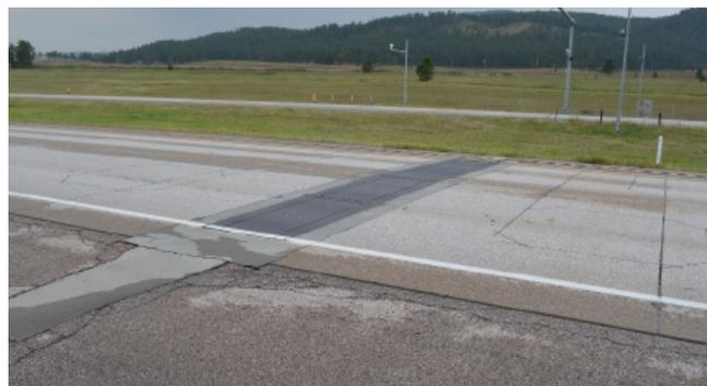
Figure 12: I-90 Traffic Data Collection Loops & Scales
