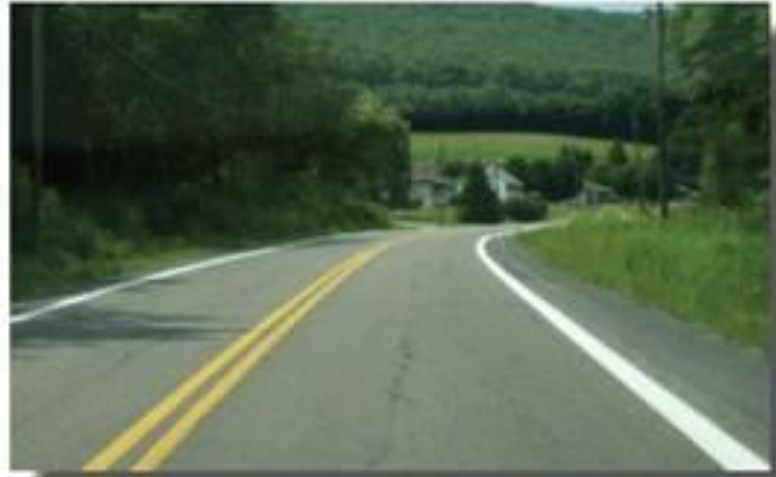
Roadway with 8-in edge line
