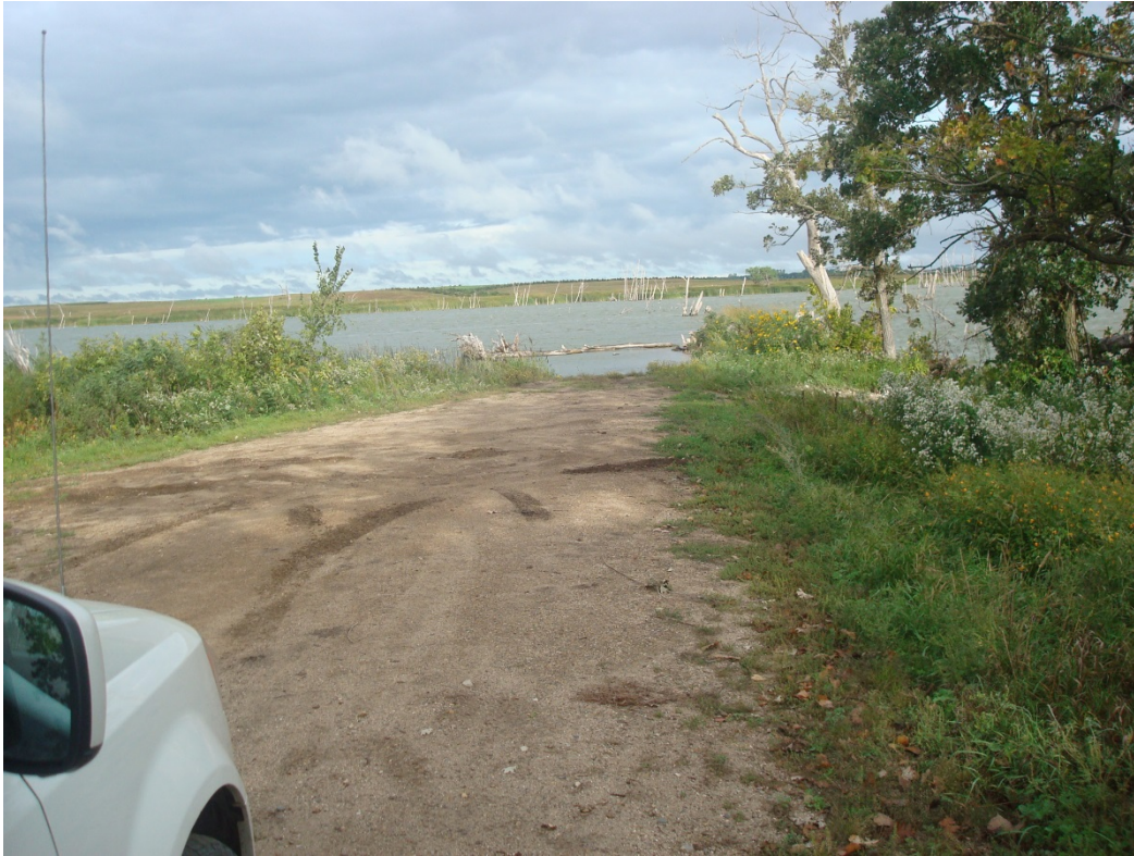
124 th Street End of Roadway at Water's Edge
