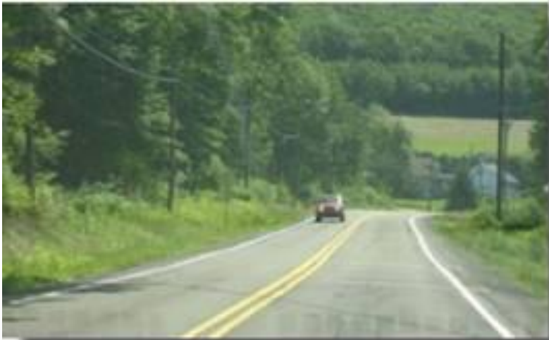
Roadway with 4-in edge line
