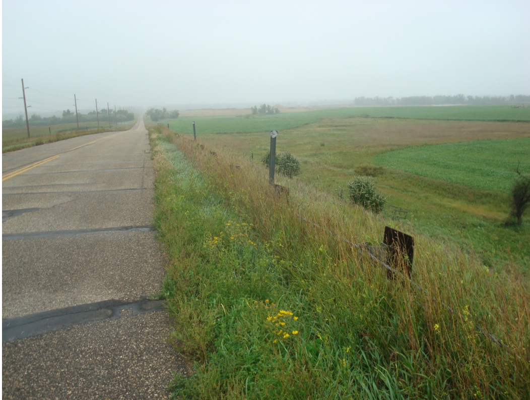
455 th Avenue With Low Cable Guardrail
