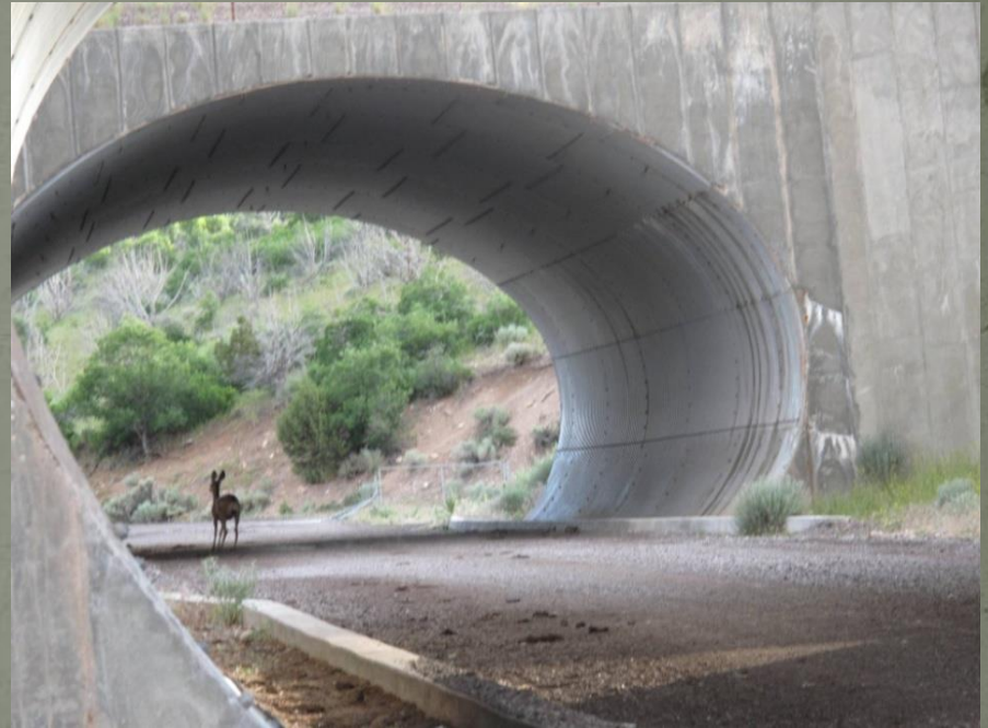
Utah I-15 Wildcat Wildlife Crossing Culvert
