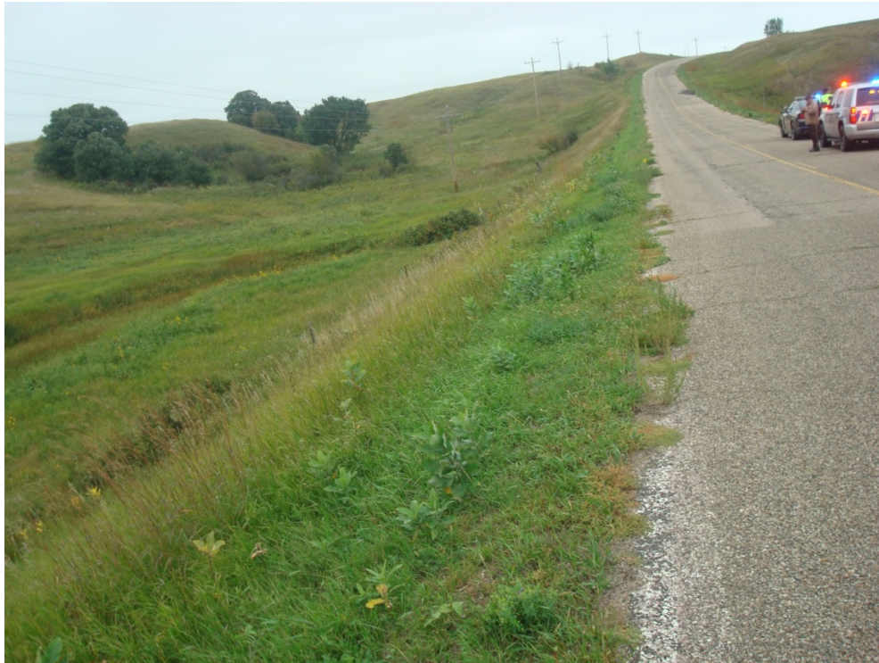
Big Lake Road No Shoulders and Steep Slopes
