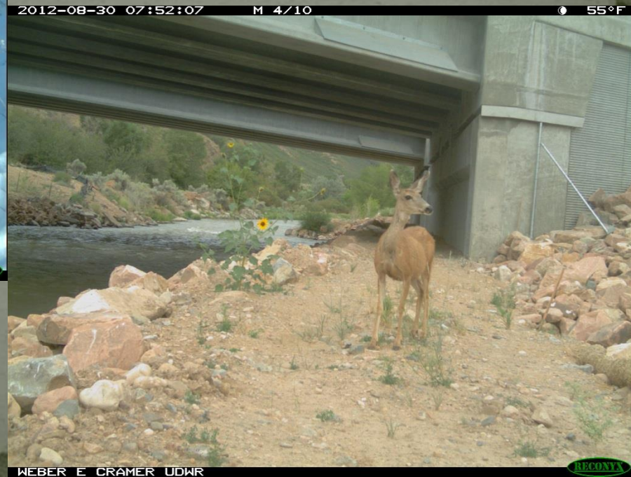
UT I-80 Weber River Bridge
