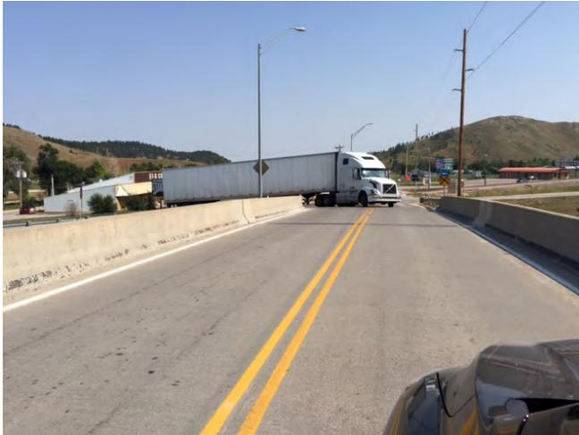
In addition, the skew of the interchange creates conflicts between vehicles on the bridge and semi-tractor trailer turning movements at the ramp terminal/service road intersections, as depicted in the photo on the left (photo credit: A. Olson, September 2015).
