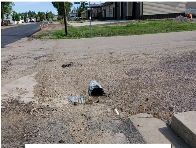
Exposed pipe culvert near intersection
