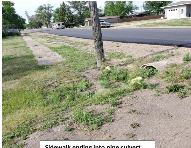
Sidewalk ending into pipe culvert
