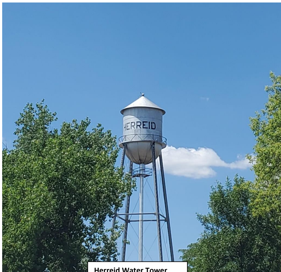
Herreid Water Tower
