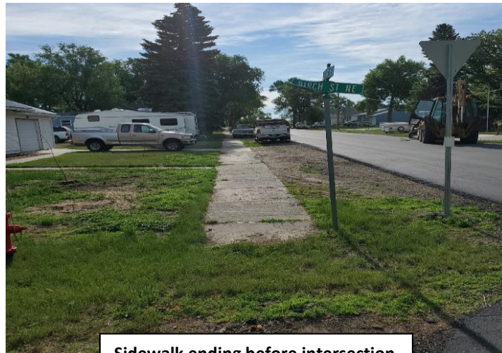
Sidewalk ending before intersection
