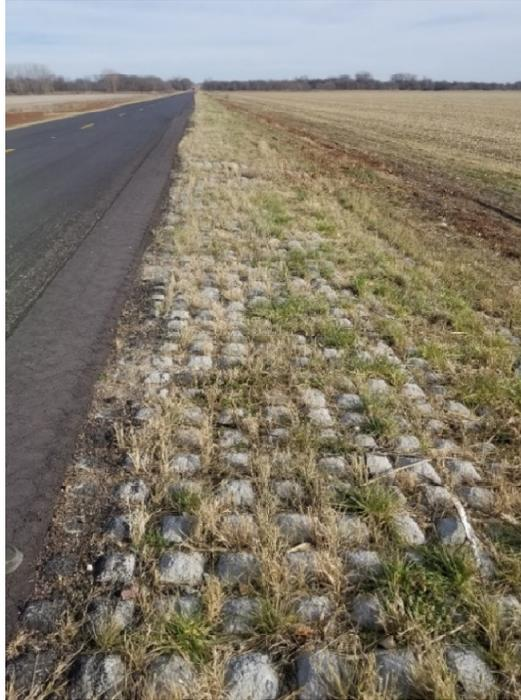
***Image of floodway with reinforced shoulders in nearby Clay County, SD***
