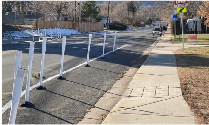
*A Quick-Build Traffic Calming Concept using flexible delineators, slows traffic in advance of a crossing
