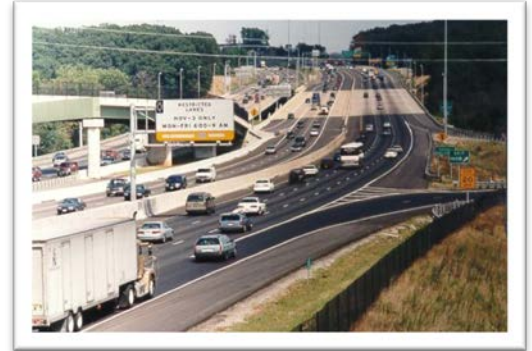
Figure 1-2: HOV Lane on Interstate 95 in Woodbridge, VA
