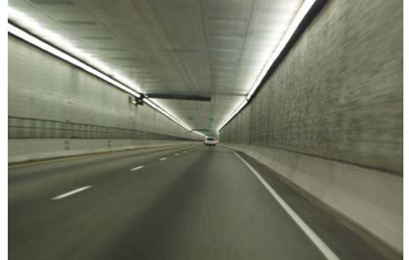
Figure 2-2: View from Inside the Eisenhower Tunnel
