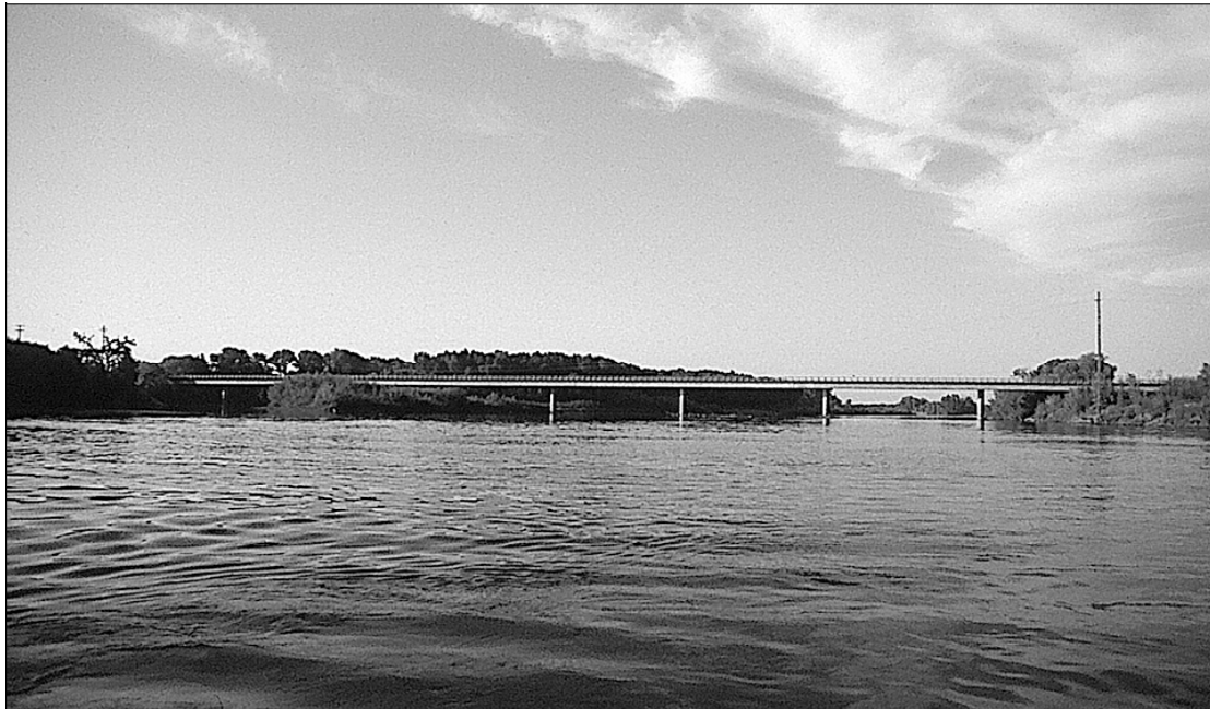
Figure 14.A-B — BRIDGE VIEW (Looking Upstream)
