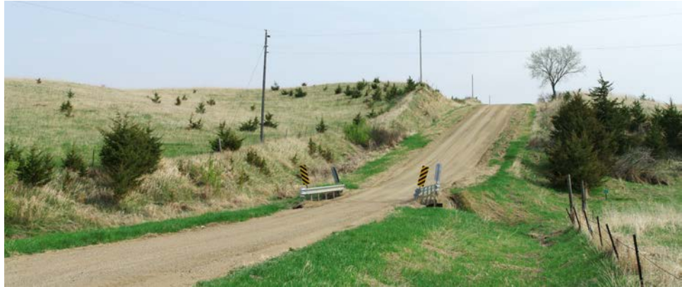
Bridge over Creek along 438 th Avenue
