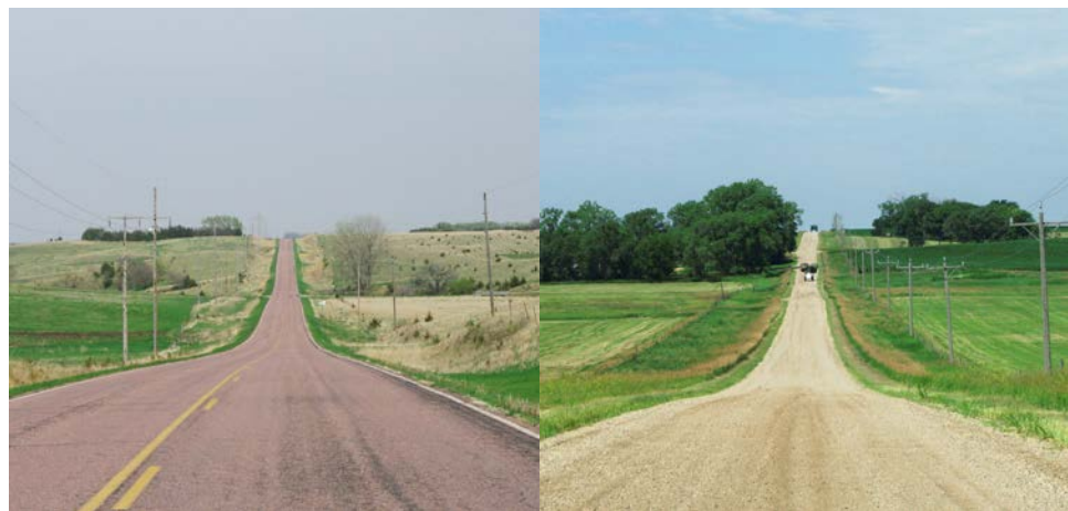
Asphalt and Gravel Roads in Yankton County
