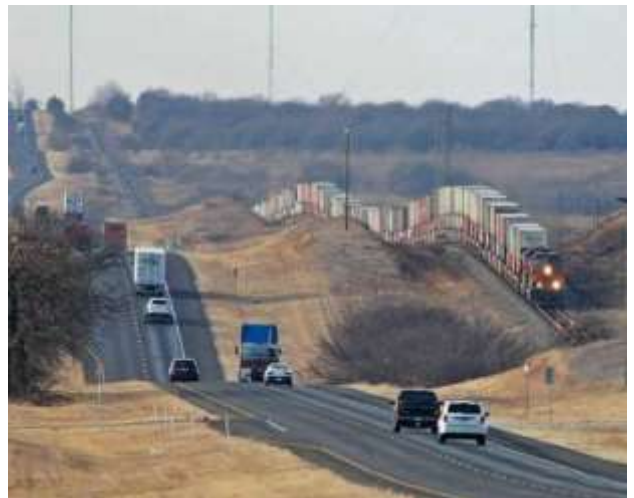
Photo 4. Example of a vertical curve in a roadway.
