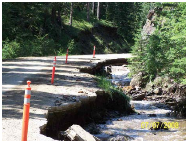
Photo 1. Example of Erosion on South Rochford Road
