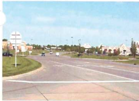
Corridor preservation can set aside land along a developing roadway for future widening.
