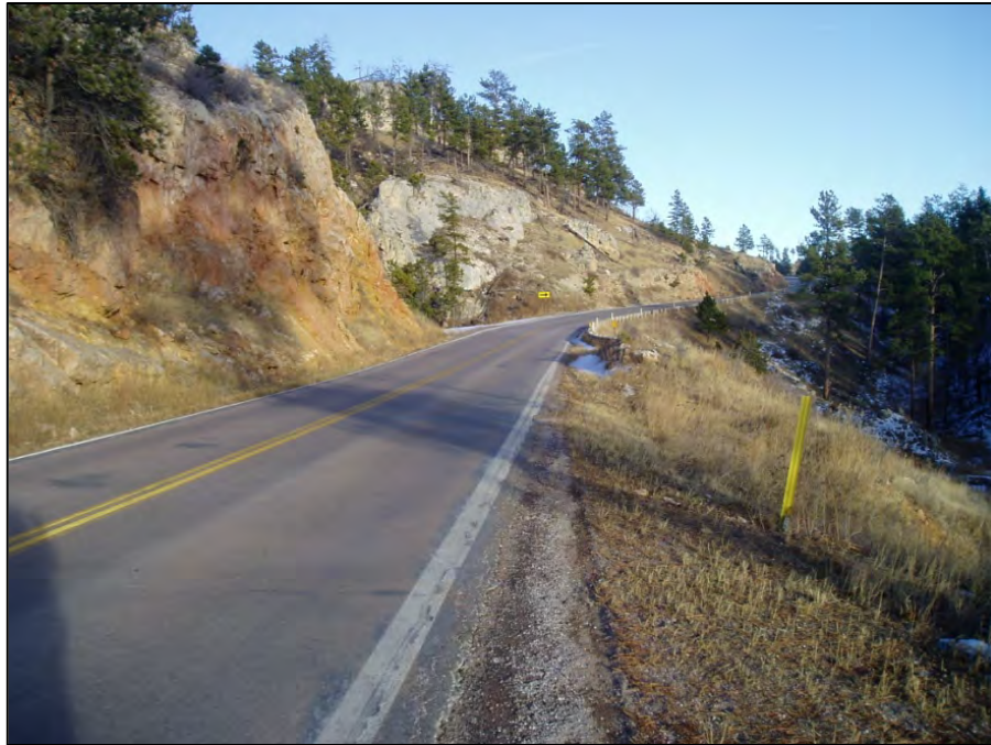
Photo 11: Photo taken facing east.
