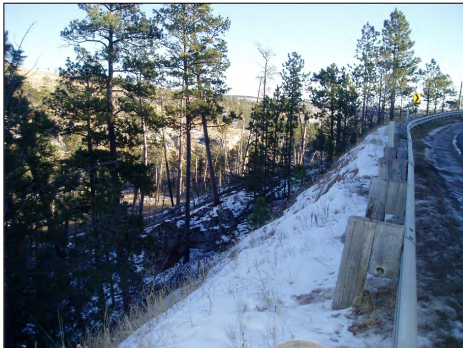
Photo 6: Photograph taken facing southeast.
