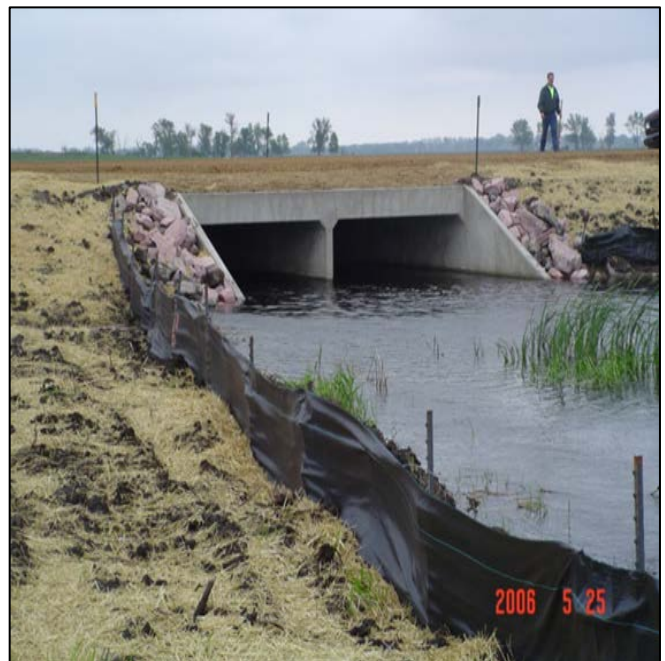
Post construction inspection of a completed structure replacement. (SDDOT)
