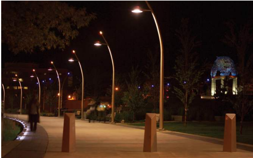
Trail lighting in Kelowna, BC © Stantec
